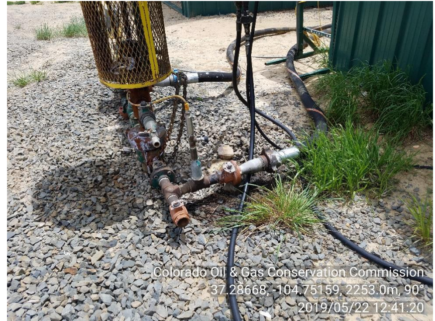
PHOTO 4: IMPACTED SOIL NEAR WELLHEAD APPEARS TO BE COMING FROM LEAKING HYDRAULIC HOSE OR HOSE QUICK CONNECT. Remove and dispose impacted material in approved manner, service and maintain equipment and self inspect to prevent recurrence of conditions per 1002.f(2) and 907" CA DATE 6/22/19
