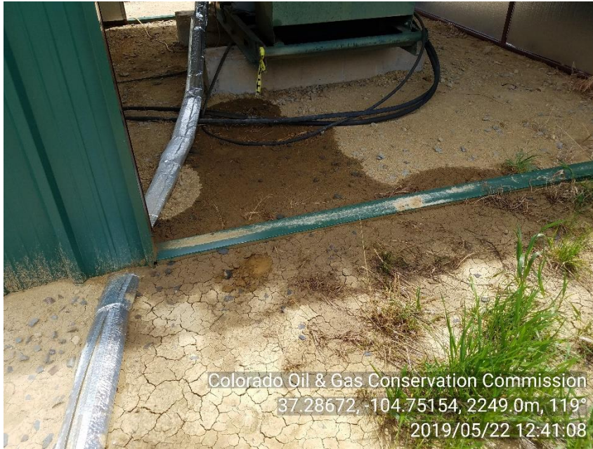
PHOTO 3: IMPACTED SOIL ON WEST SIDE OF PRIME MOVER ENGINE SKID. Remove and dispose impacted material in approved manner, service and maintain equipment and self inspect to prevent recurrence of conditions per 1002.f(2) and 907" CA DATE 6/22/19
