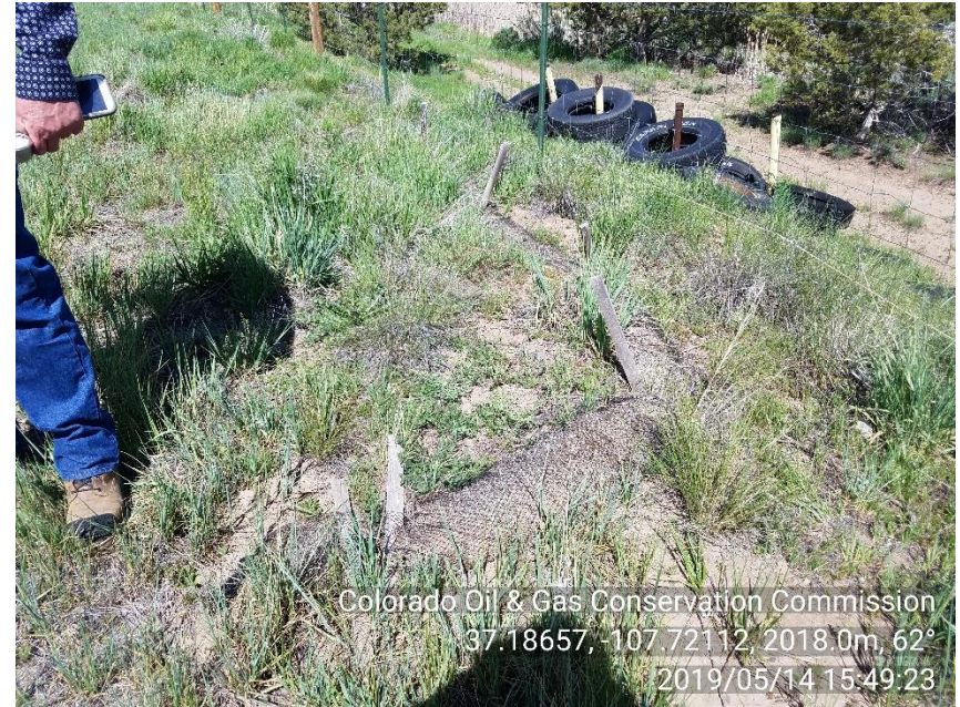
PHOTO 8: REMOVE OR REPAIR BMP WADDLES ON EAST SIDE OF LOCATION. Install or repair required BMPs per Rule 1002.f. CA DATE 6/14/19
