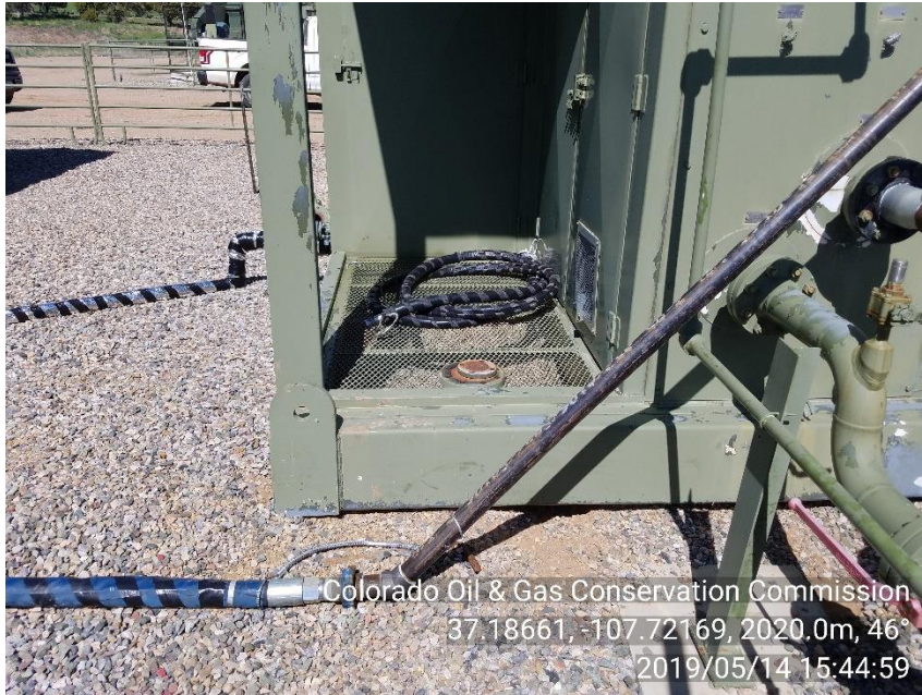
PHOTO 9: UNUSED EQUIPMENT HOSE ON SEPARATOR SKID. COMPLY WITH RULE 603.f. CA DATE 6/14/19
