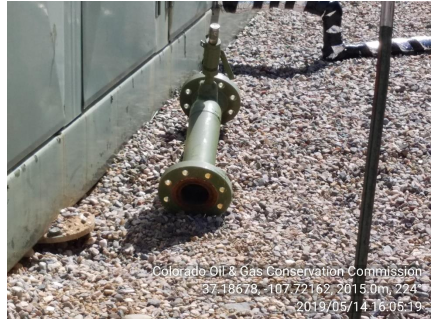
PHOTO 9: UNUSED EQUIPMENT PIPE SUB ON LOCATION NEAR SEPARATOR HOUSE. COMPLY WITH RULE 603.f. CA DATE 6/14/19
