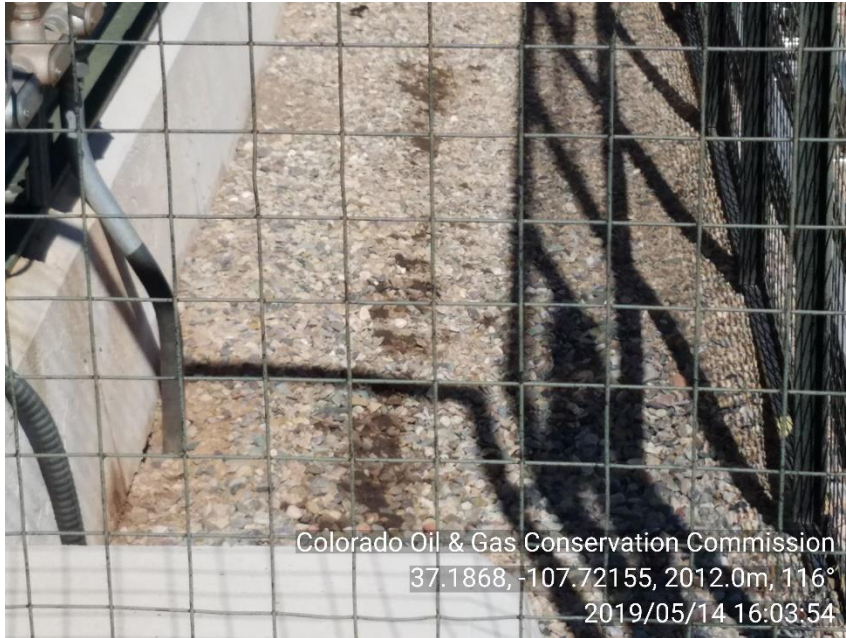
PHOTO 5: IMPACTED SOIL NEAR EAST SIDE OF PUMPJACK. Non E&P Waste not properly stored, handled, transported, treated, or disposed per Rule 907A. CA DATE 6/14/19
