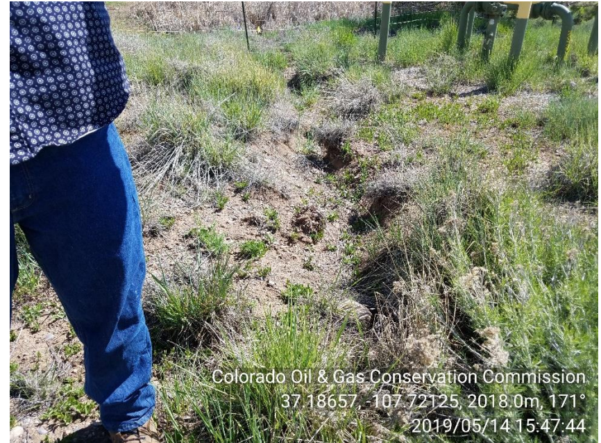
PHOTO 6: EROSION ON EAST SIDE OF LOCATION. Install or repair required BMPs per Rule 1002.f. CA DATE 6/14/19
