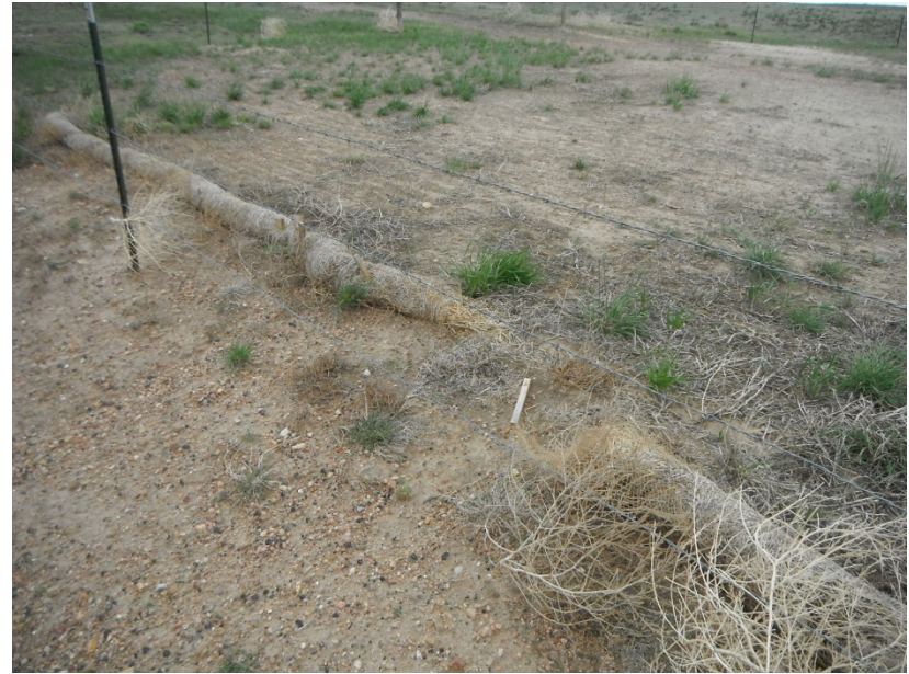
Damaged straw waddles
