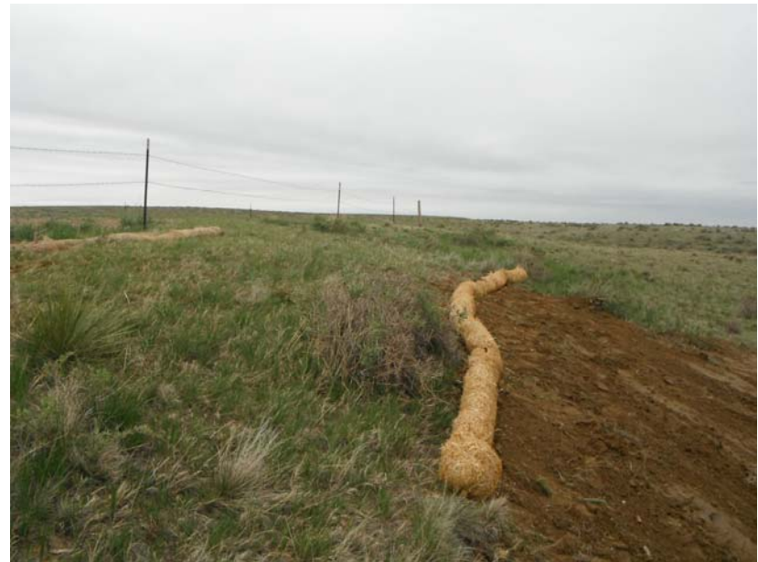
Additional straw waddle above west eroded area
