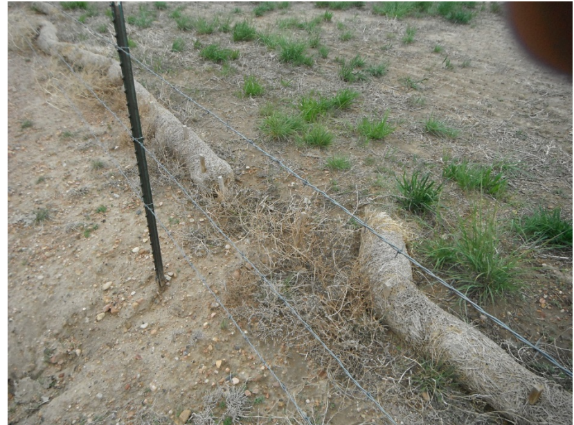
Damaged straw waddles
