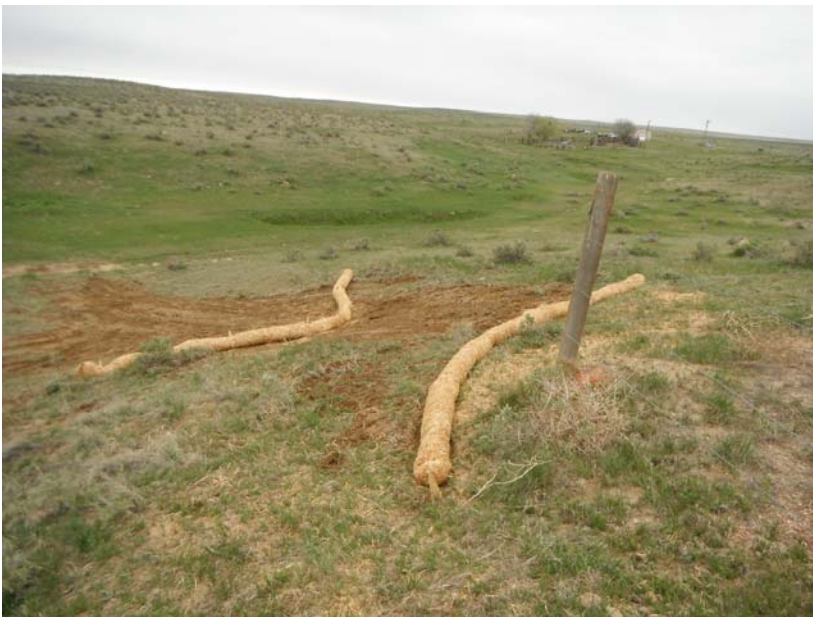
Northwest channel after regrading and repairs
