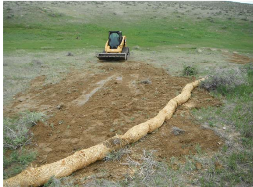
West eroded area after regrading and waddle placement
