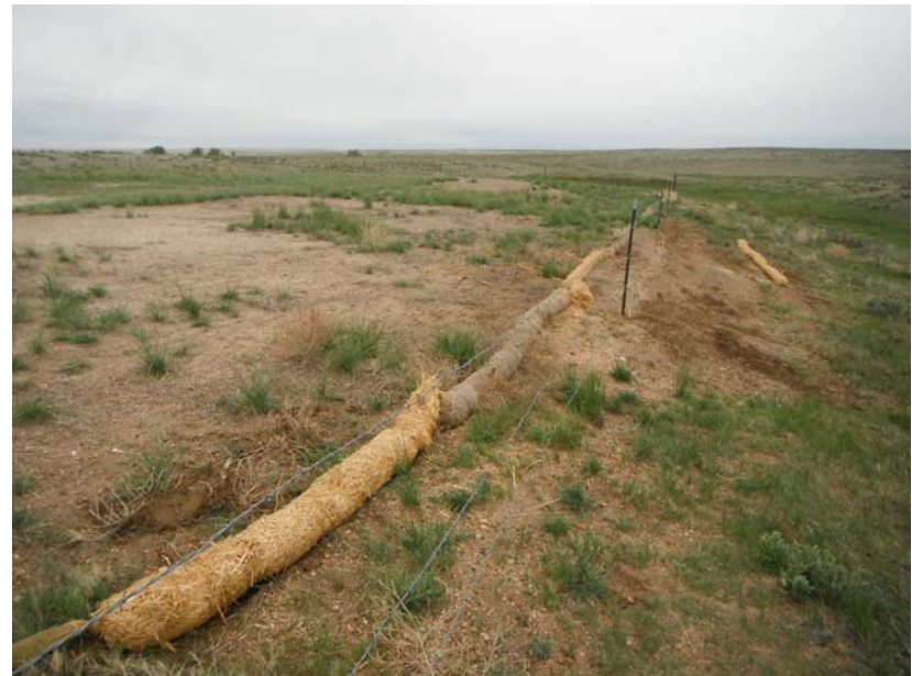
Repaired straw waddles on north side with extra waddle
