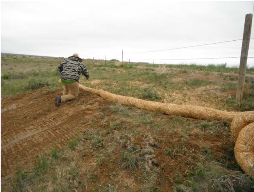
Placing straw waddle at northwest corner
