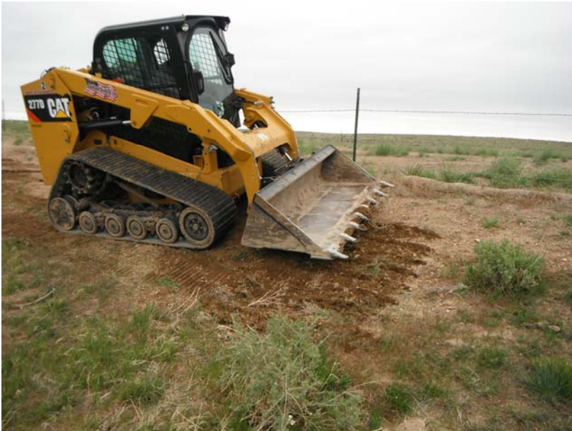
Regrading north erosional channel
