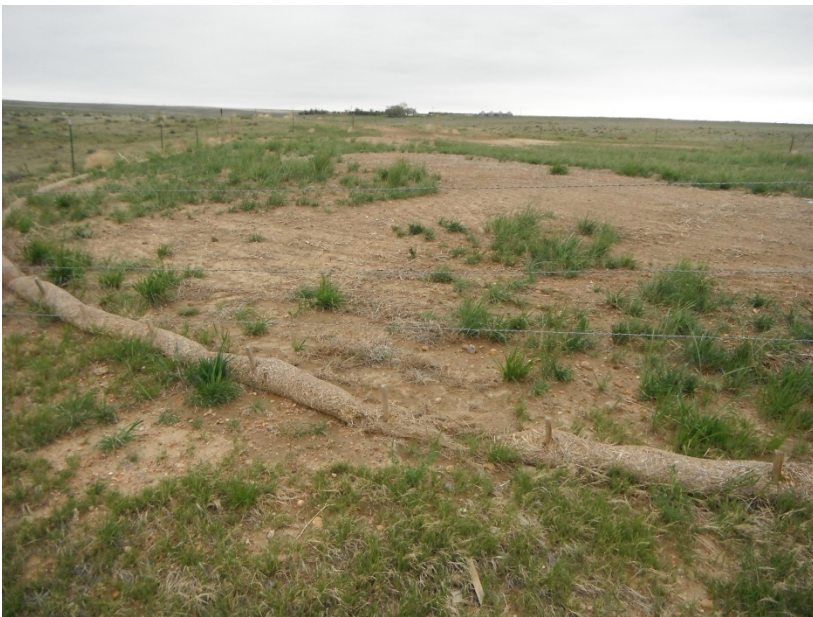
Damaged straw waddles
