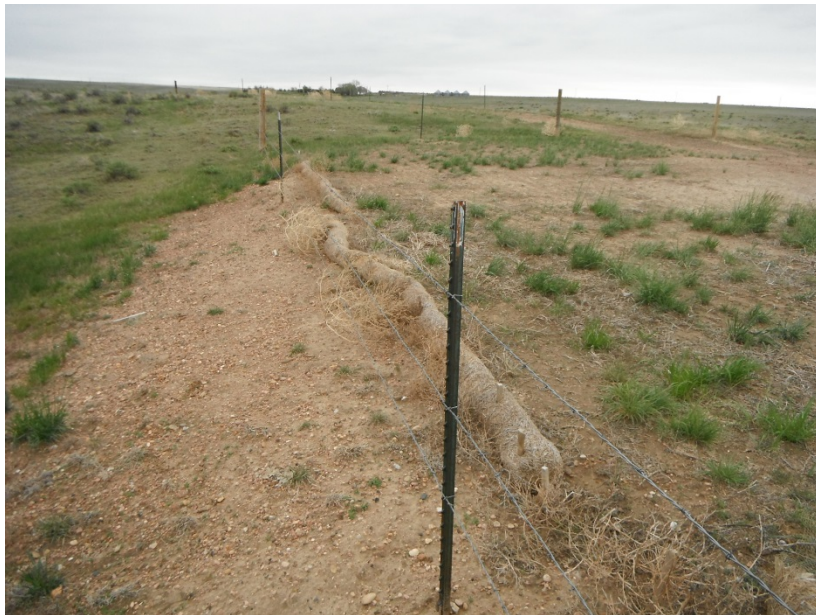
Damaged straw waddles on north side of former well pad
