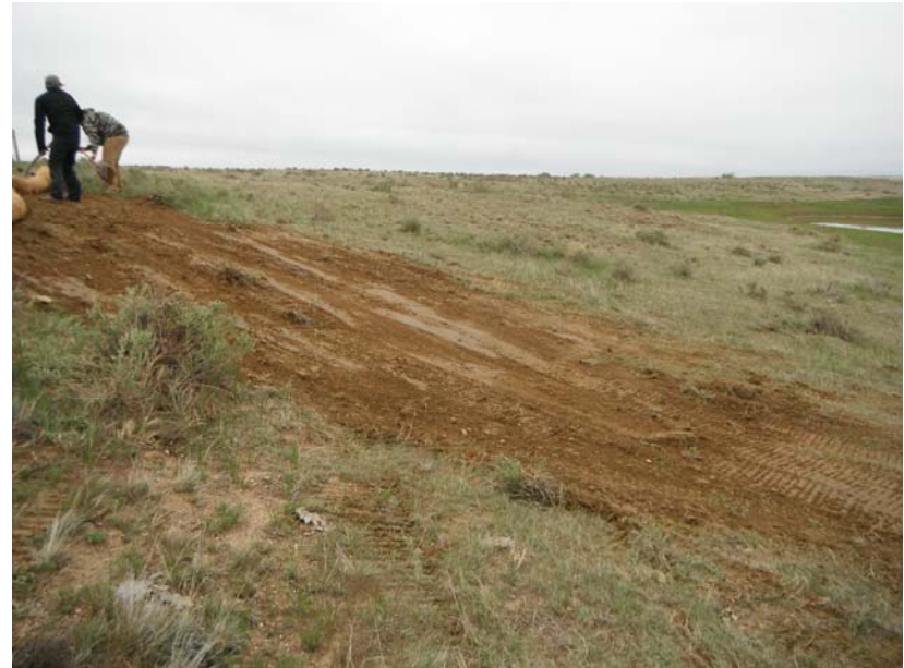
Regrading the west eroded area and placing waddle
