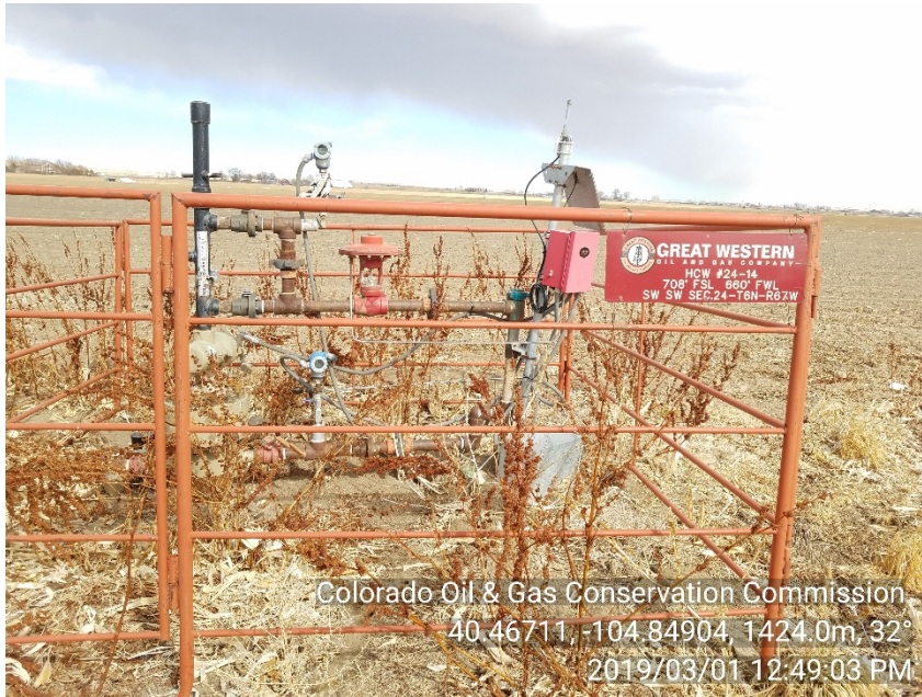
Photo #5 HCW 24-14 (05-123-31498) Wellsite Shut-In | SI Emergency number NOT posted Weeds from prior insp.
