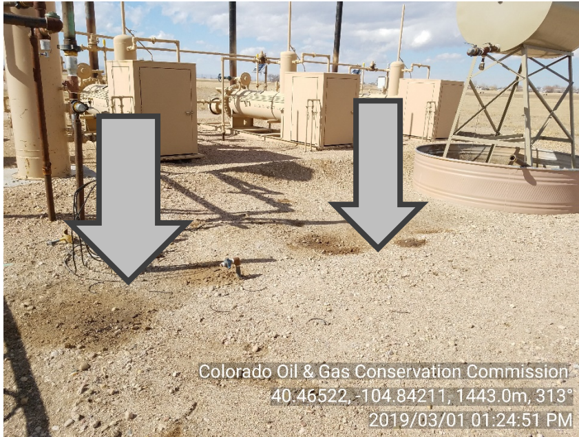
Photo #3 Battery HCW 23-43, 23-54 HCW 24-24, 24-13, 24-14, 24-23, 24-53 HCW FD 24-20D, 24-35D, 24-36D Stained soil – from prior insp.
