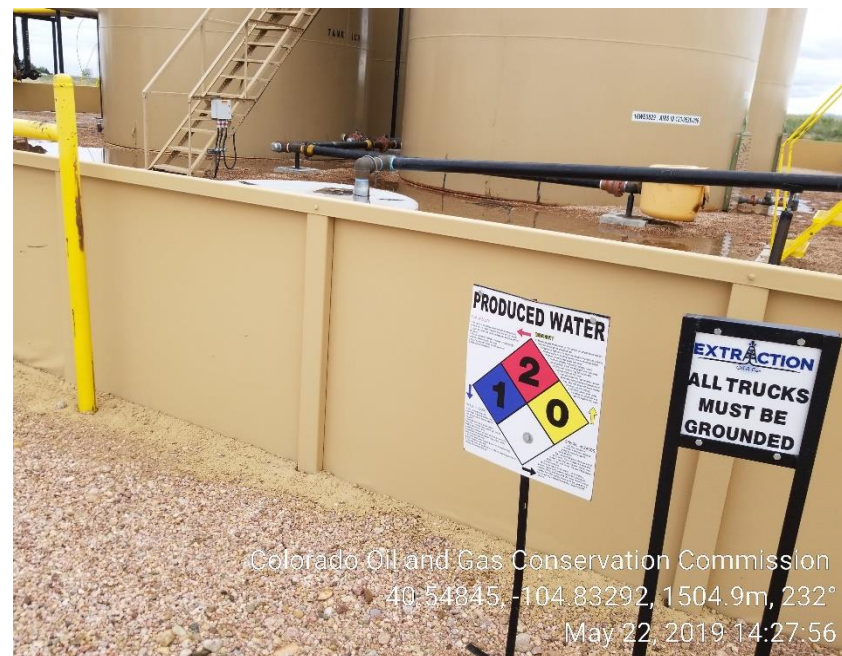
Photo 14: No BBLS listed on Produced water tank.
