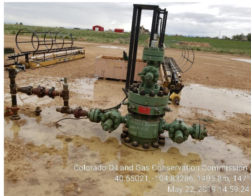
Photo 8: (TA) Wellhead; NO SIGN, UNUSED EQUIPMENT
