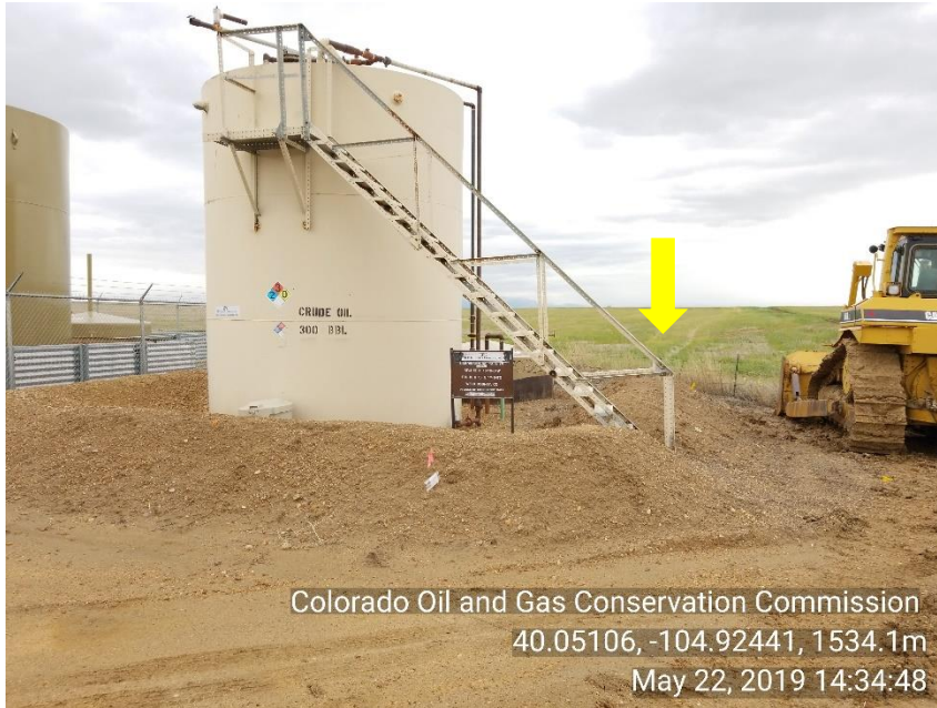
Photo 5 TNk BTRY. Inadequate berms material appears to be pushed up and dot compacted.
