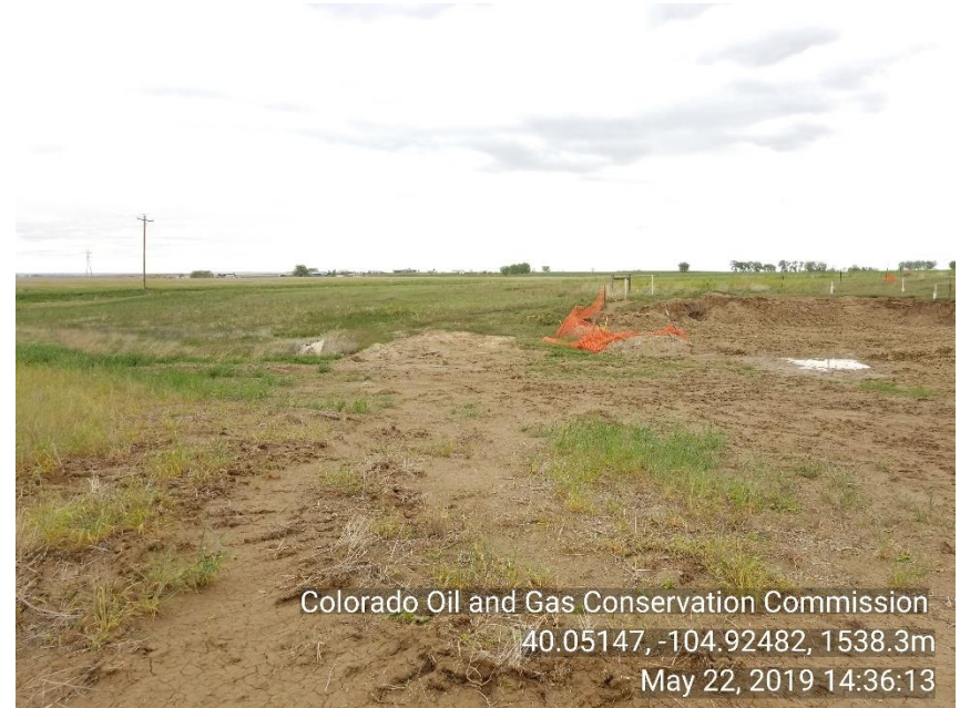
Photo 8 excavation safety fence in disrepair. No BMP's in place of excavation.
