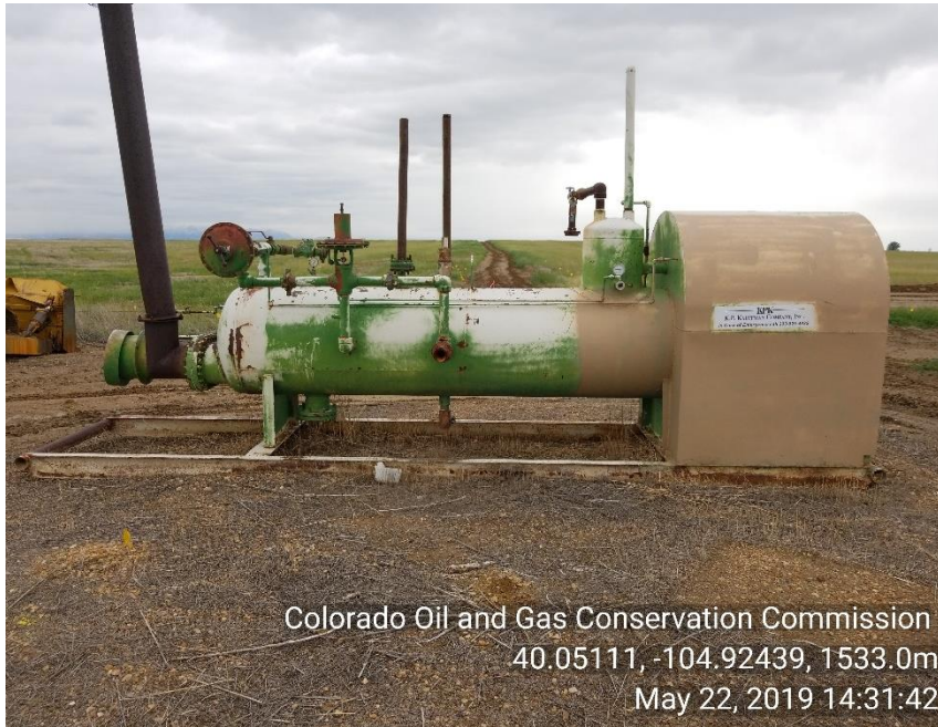
Photo 1 Unused equipment: Separator, appears all flow line piping has been removed.
