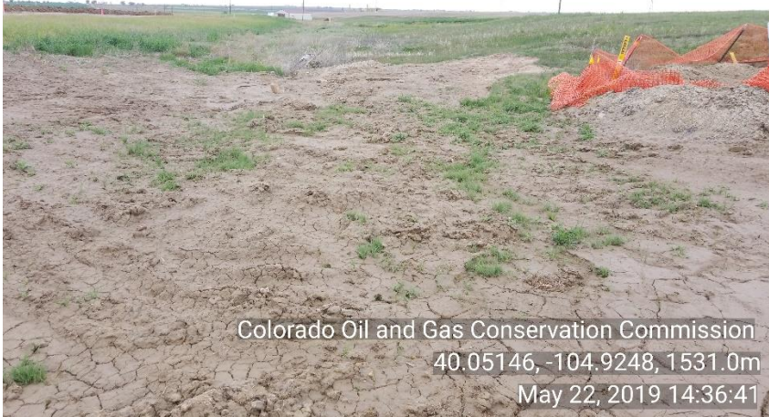
Photo 9 No BMP's controlling sediment from running off excavation. Sediment being carried down natural drainage. Safety fence in disrepair.
