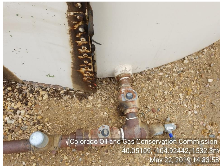
Photo 4 flow lines to tank valves are closed
