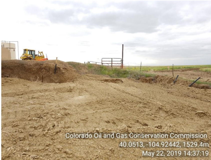
Photo 11 Several flow lines exposed, no BMP's in place around excavation. No safety fence around open excavation.
