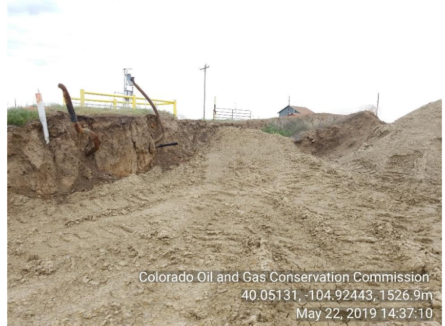
Photo 10 Several flow lines exposed, no BMP's in place around excavation. No safety fence around open excavation.
