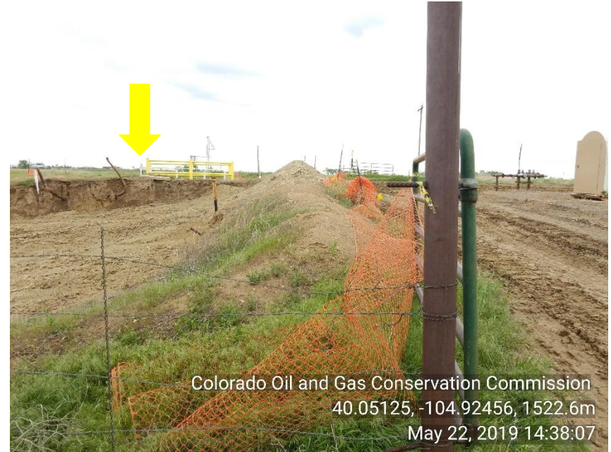
Photo12 Safety fence in disrepair. No BMP in place on open excavation for run on.
