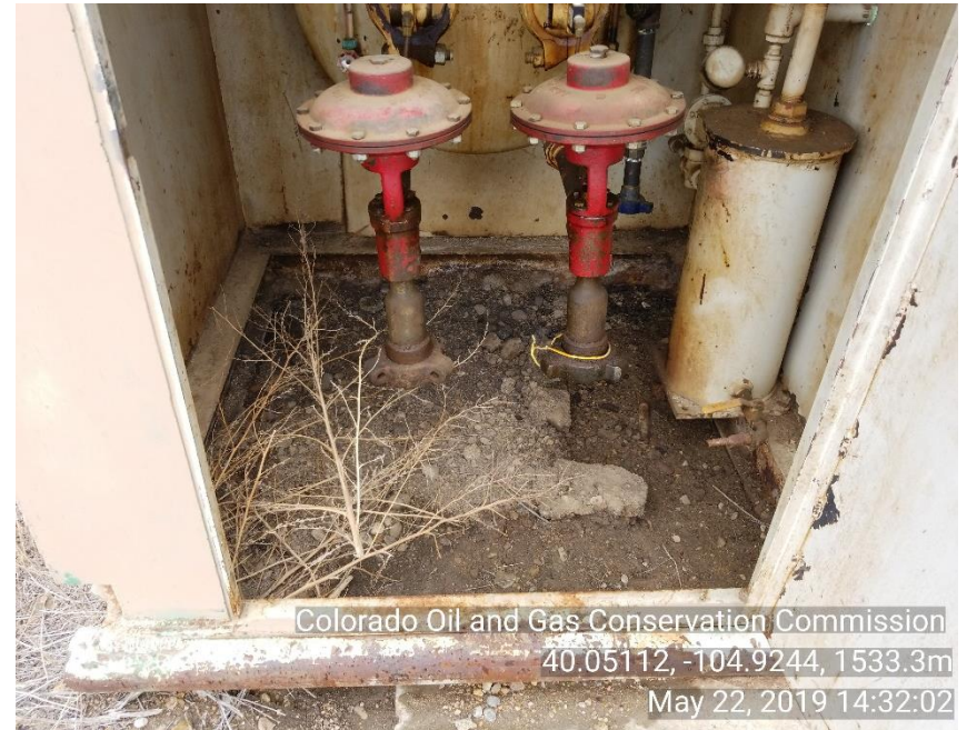
Photo 2 Unused equipment: Separator, appears all flow line piping has been removed.
