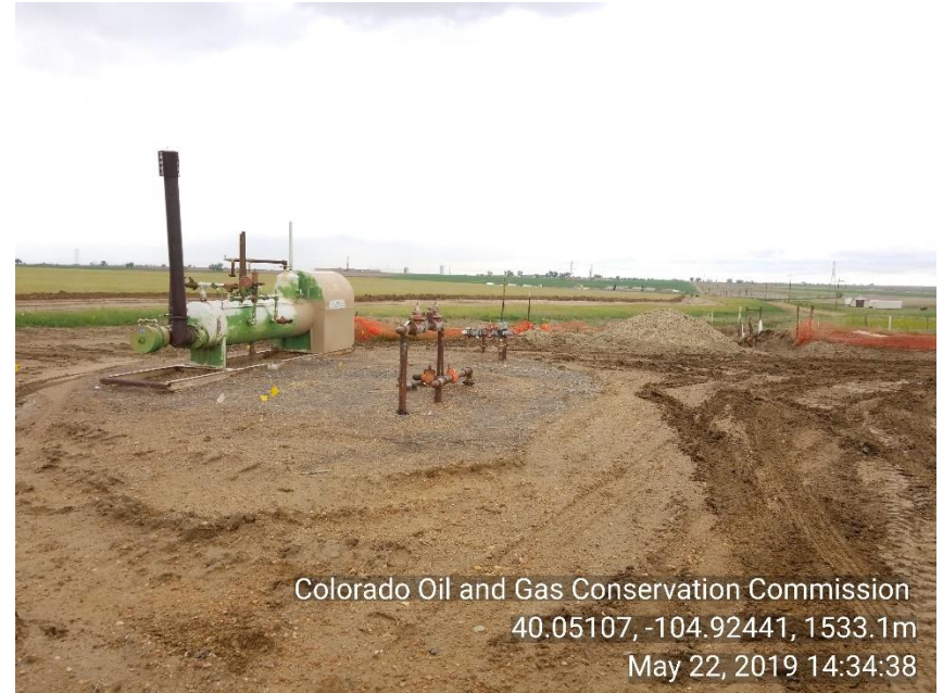
Photo 6 loc pic. Spoil piles with out BMP's, Safety fence in disrepair.
