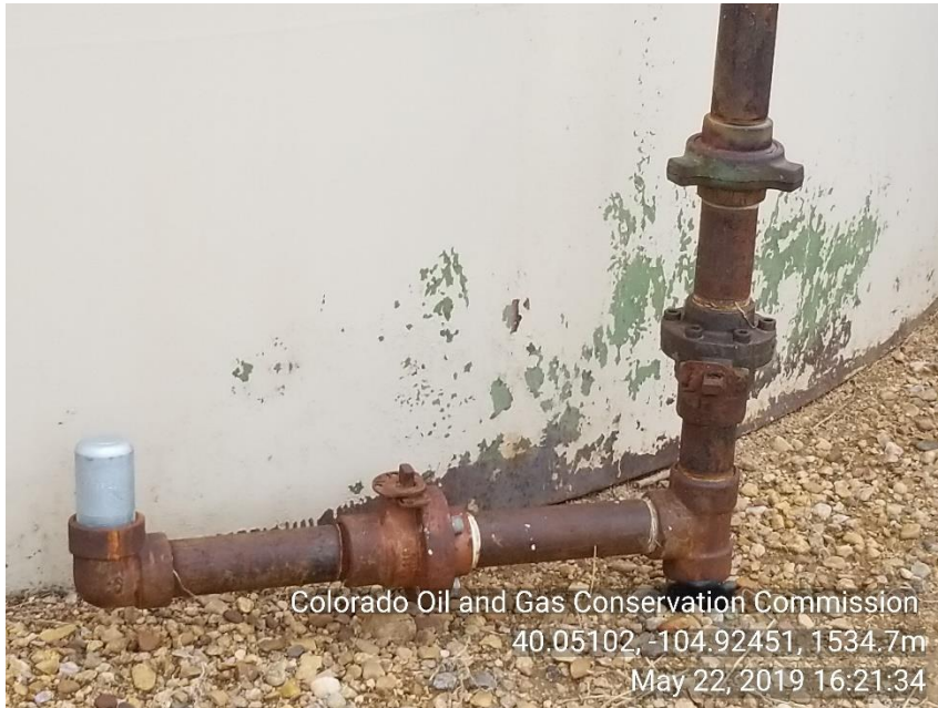
Photo 7 flow line valves to crude oil tank closed
