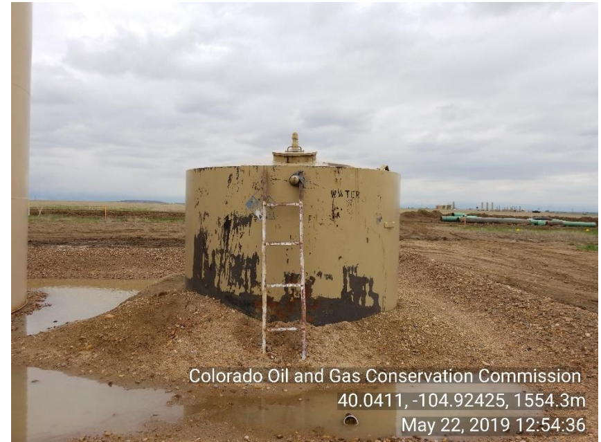
Photo 6 No NFPA placard and no tank volume on produced water tank.
