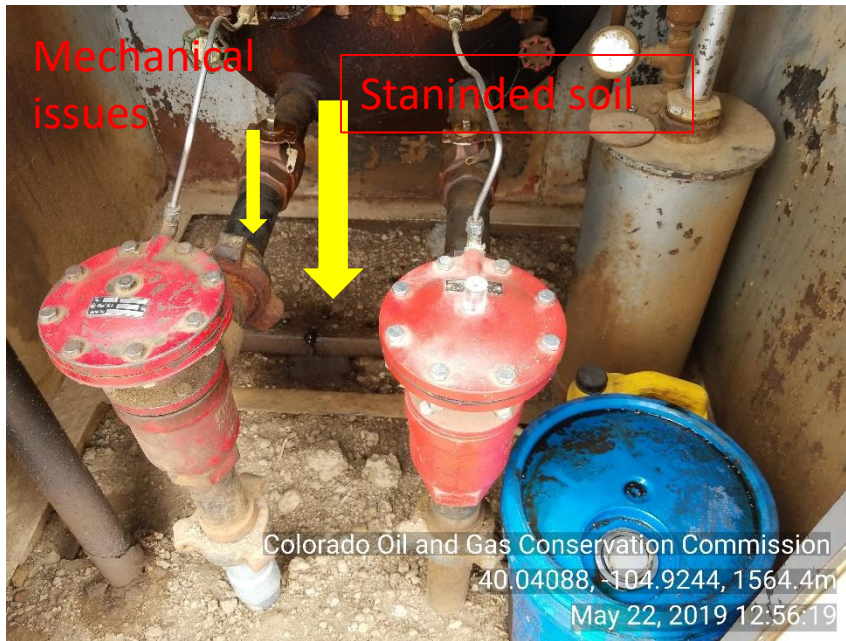
Photo 9 Trash: 5 buckets. Stained soil, Mechanical issues appears piping is leaking on ground.
