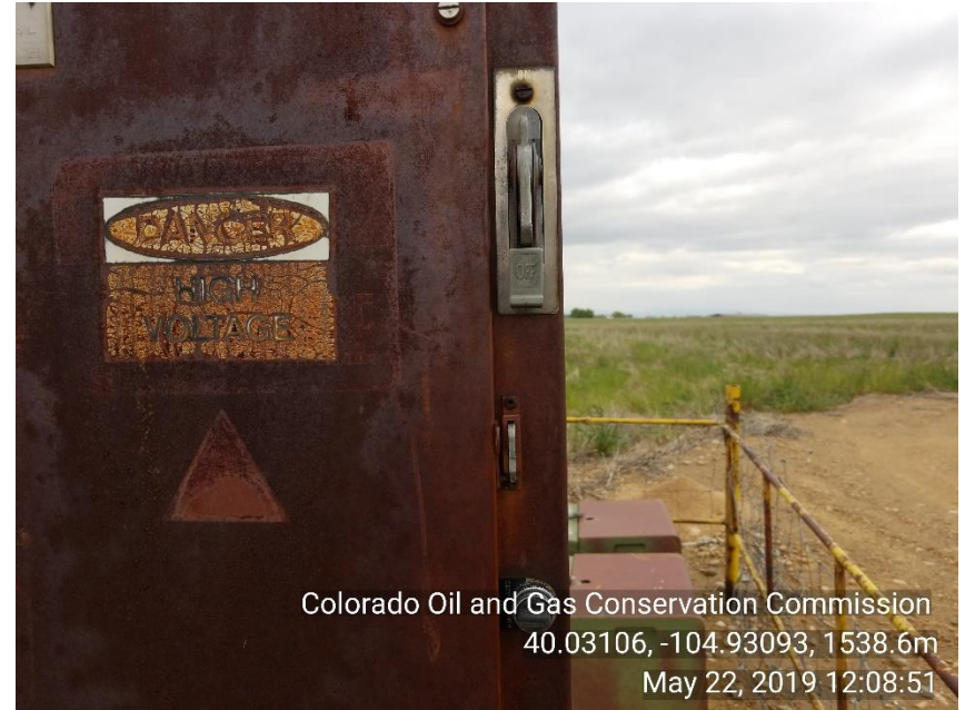
Photo 4 Electric power to PU is in the off position at breaker box. Well cannot pump on timer.
