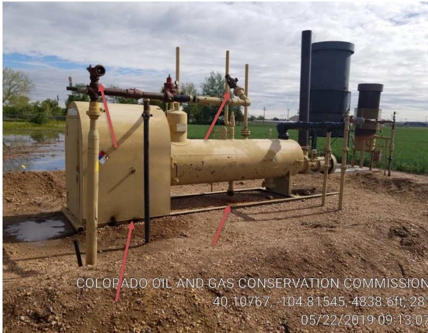
Pic 1 separator lines not plugged.
