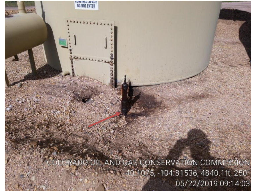
Pic 2 stained soil possible leak on oil tank
