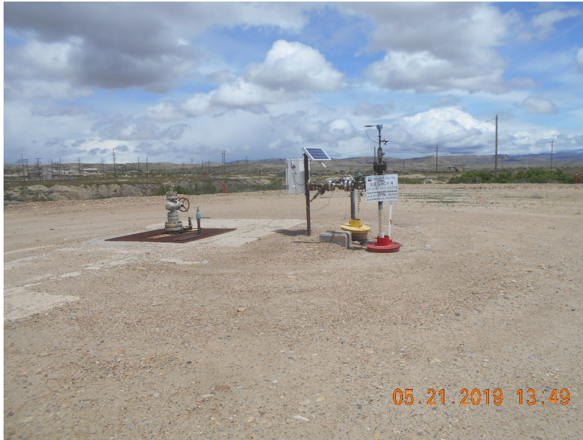
Injection wellhead
