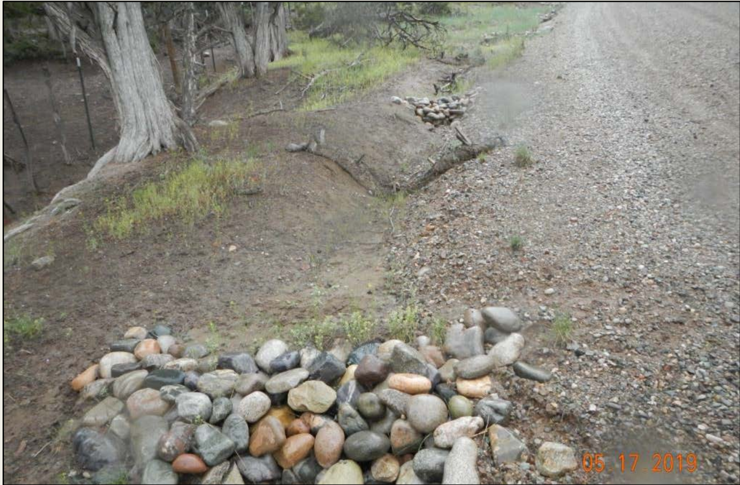
Photo 3. View of stormwater controls along the access road that are full of sediment and need maintenance.
