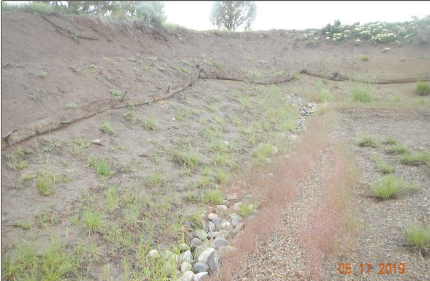
Photo 2. View of cut-slopes in the northwestern project area that are not stabilized.
