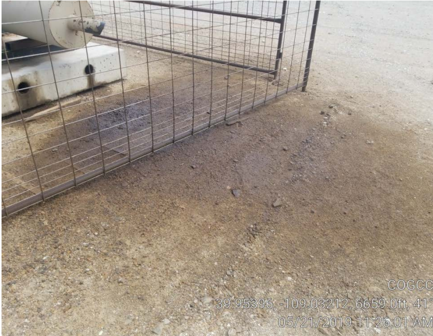
Photo 2. Oily waste on ground at pump jack exhaust.
