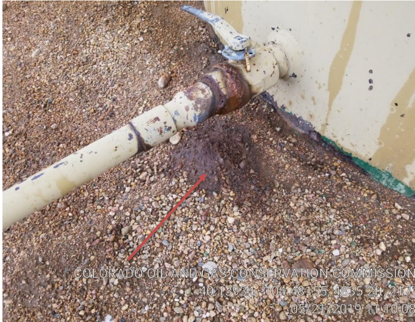
Pic 5 stained soil under valve
