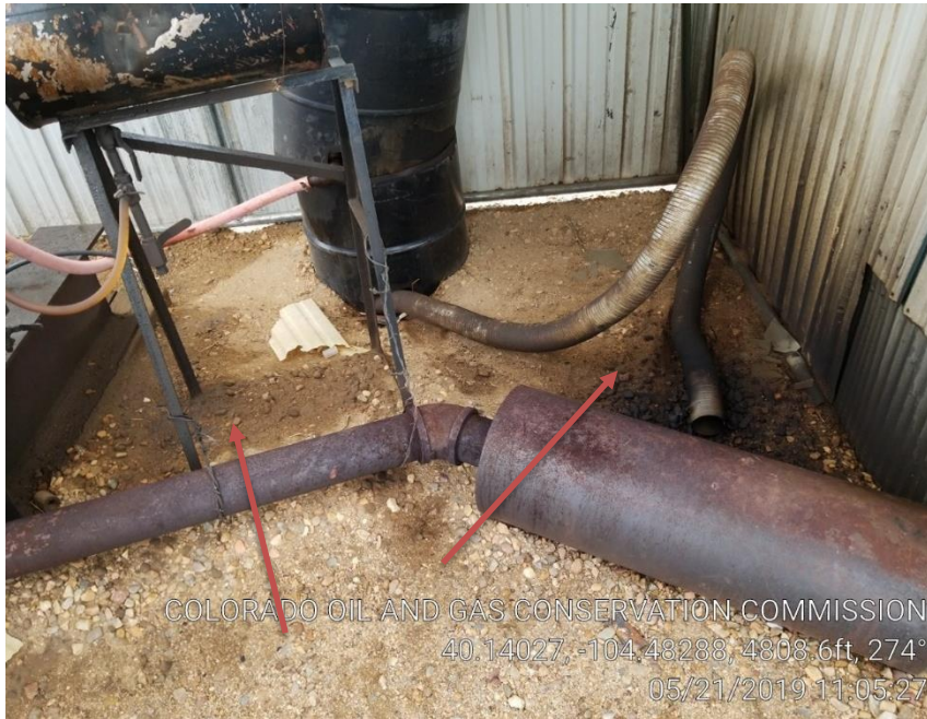
Pic 3 stained soil in motor house
