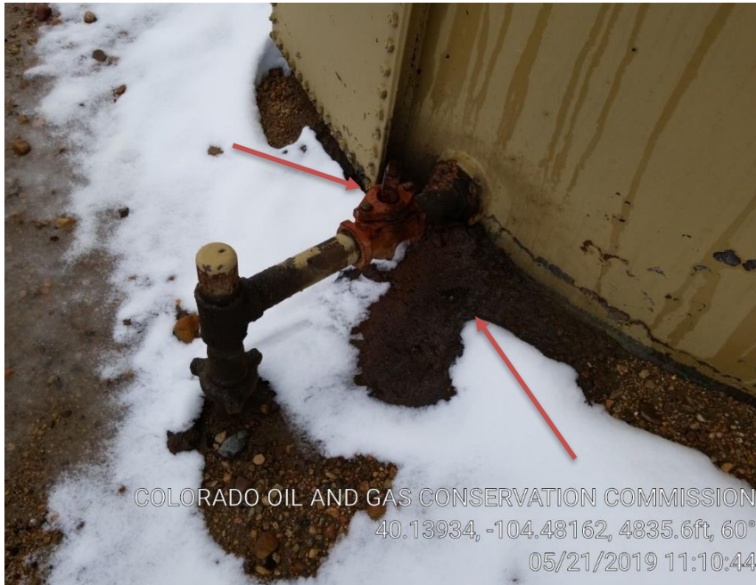
Pic 7 leaking valve behind tank
