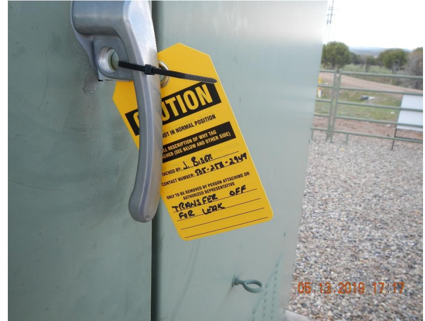
Locked out/tagged out equipment as a result of Spill/Release Point ID #464472.
