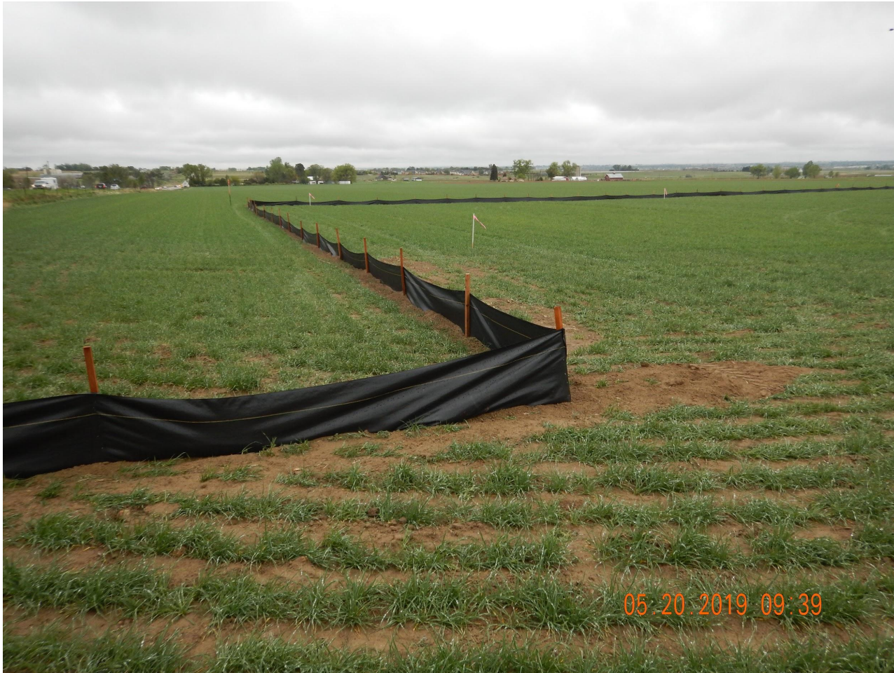
Photo 3. Photo taken from the northern location, facing East. Operator has install initial stormwater BMPs prior to the start of construction per Rule 1002.f. Note: It appears silt fence stakes have been installed too far apart. Per Rule 1002.f., Operator shall install stormwater BMPs per good engineering practices.
