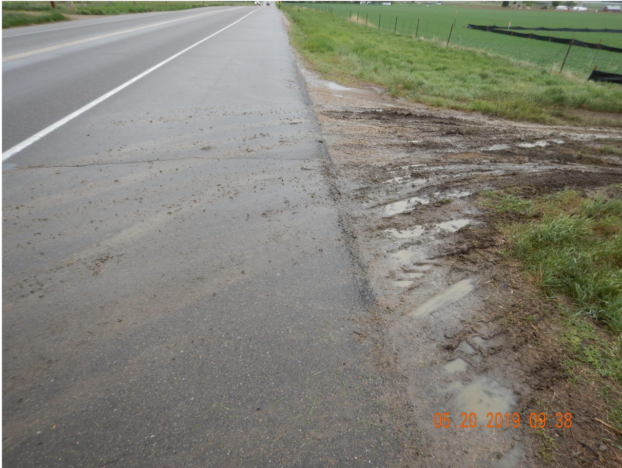
Photo 1. Photo taken from the entrance to location, facing East. Operator has failed to install a vehicle tracking device BMP. Operator is tracking out sediment and rutting up the entrance.
