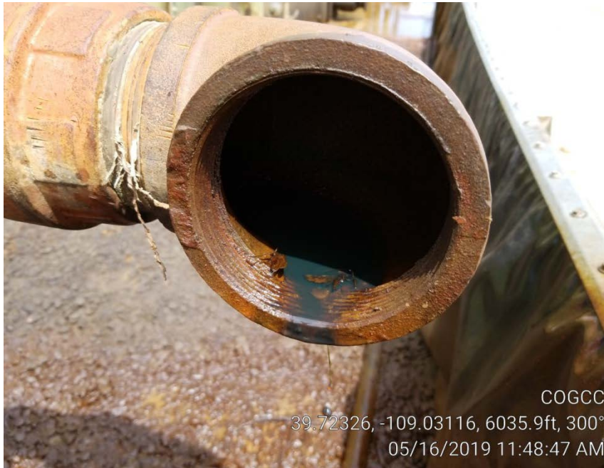
Photo 4. Condensate dripping out offload connection.
