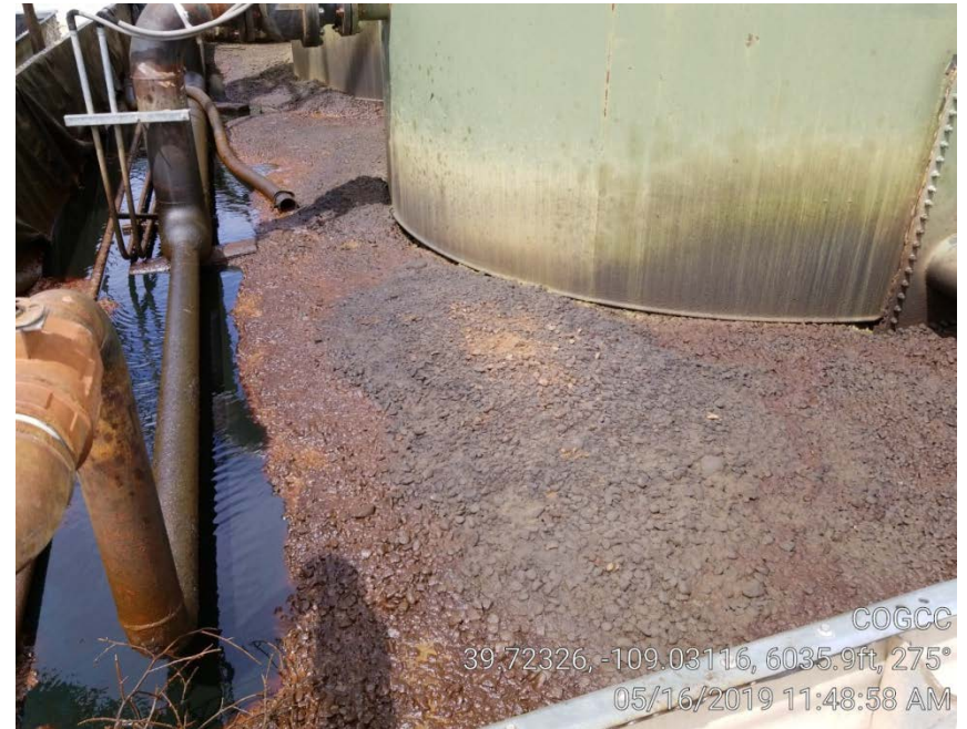
Photo 5. Gravel inside tank berm soaked with condensate.
