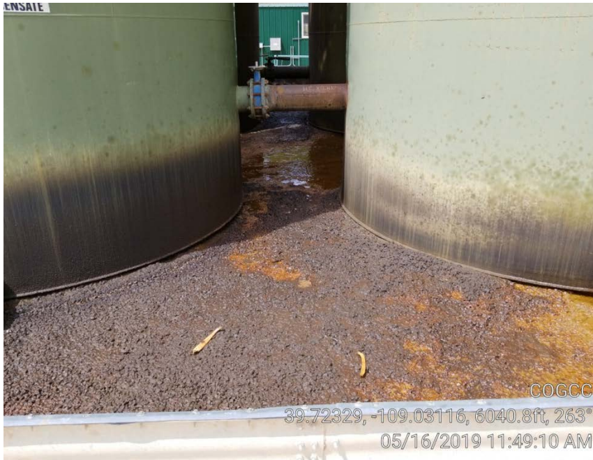
Photo 6. Gravel inside tank berm soaked with condensate.
