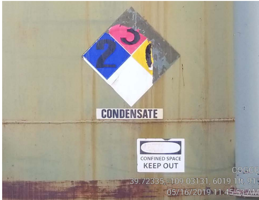
Photo 8. Tank label without capacity, operator and phone number.
