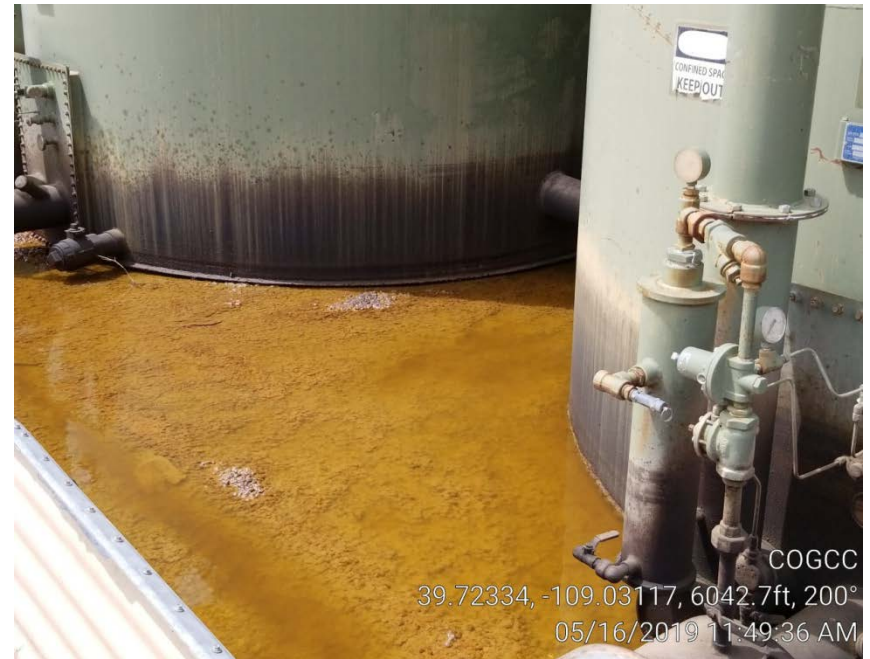
Photo 7. Condensate sheen on top of water inside tank berm.
