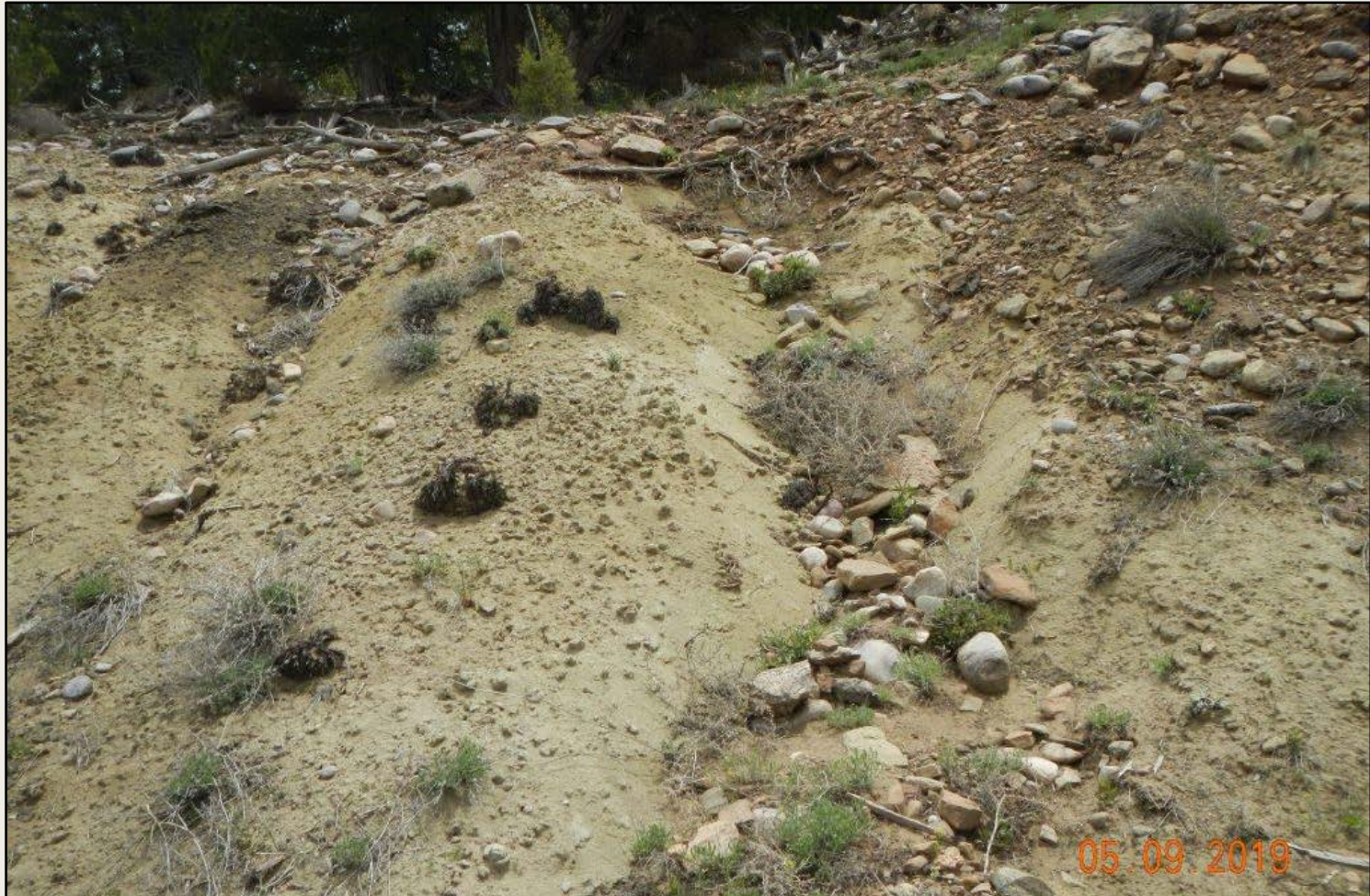
Photo 2. View of erosional channeling in the well pad cut-slope. Exposed roots, scouring, and sediment deposition indicate erosion.
