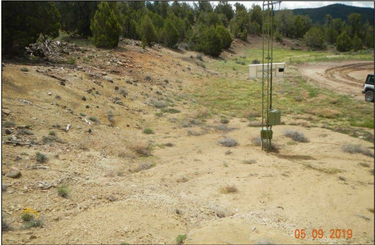
Photo 1. View of the eastern project area from the northeastern corner facing southward. Cut slopes are eroding.
