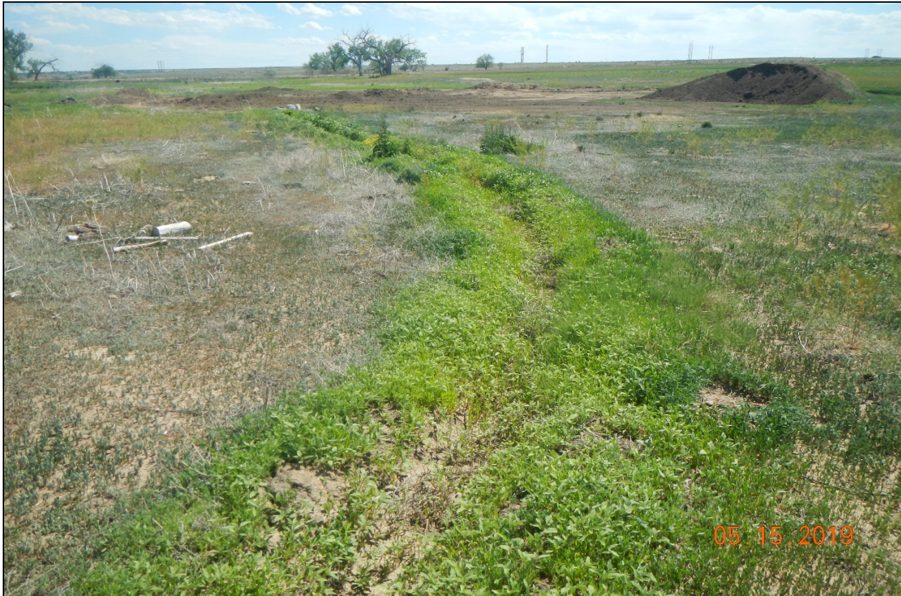
Photo 3. The ditch directed toward the pit needs to be filled and reclaimed.
