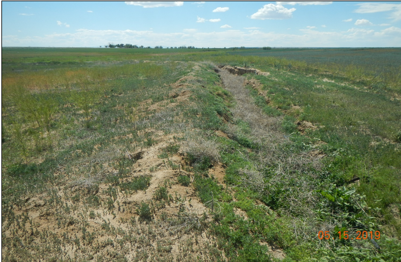
Photo 4. The ditch at the north side of the location that wraps around to the southwest must be filled in and reclaimed.
