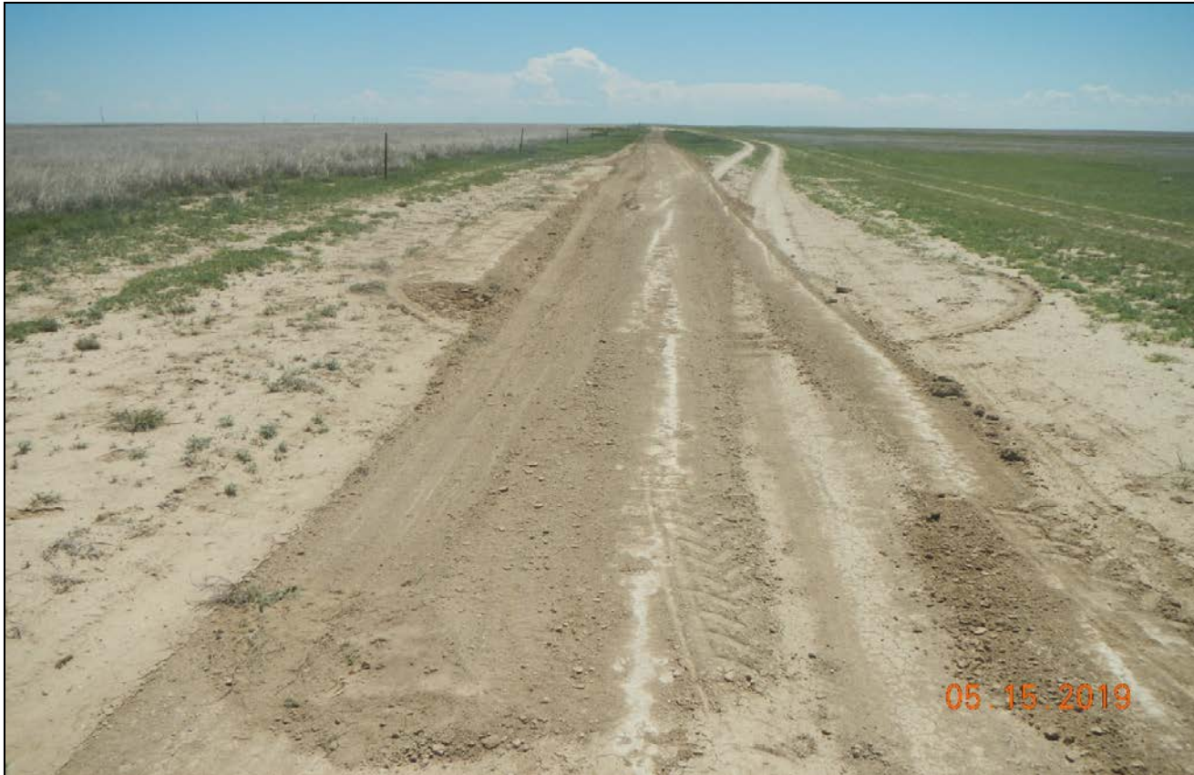
Photo 3. It appears water pools onto the access road. A new road has been made by vehicles avoiding this area when wet causing additional disturbance that needs to be reclaimed and prevented.
