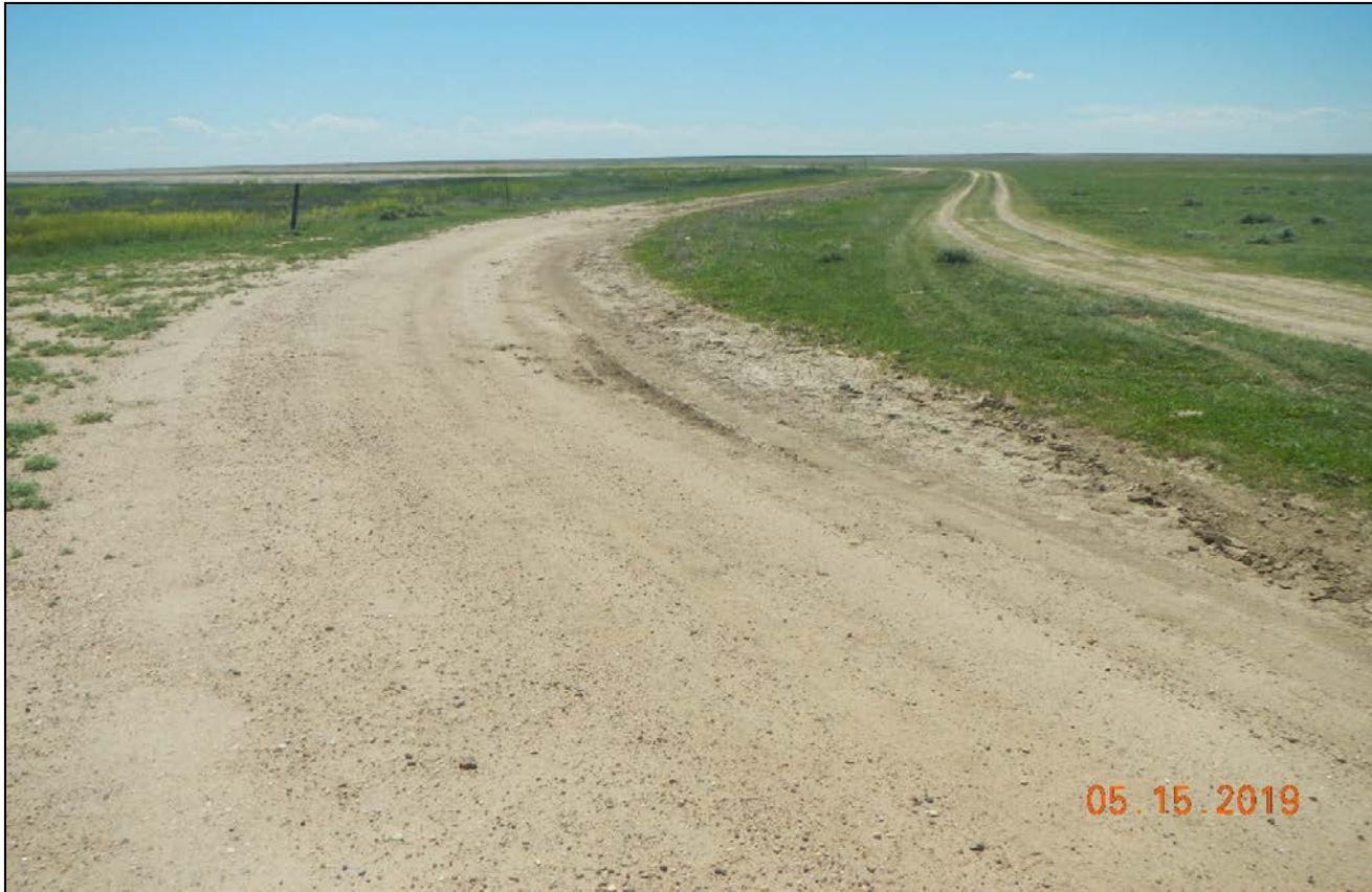
Photo 2. It appears water pools onto the access road. A new road has been made by vehicles avoiding this area when wet causing additional disturbance that needs to be reclaimed and prevented.
