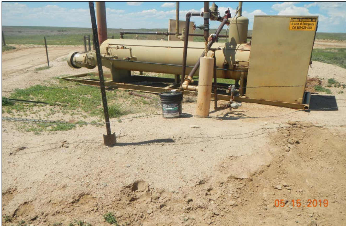
Photo 7. The berms are not sufficient the fencing around the equipment is not sufficient to prevent livestock entry. Unknown 5 gal container is stored near equipment.
