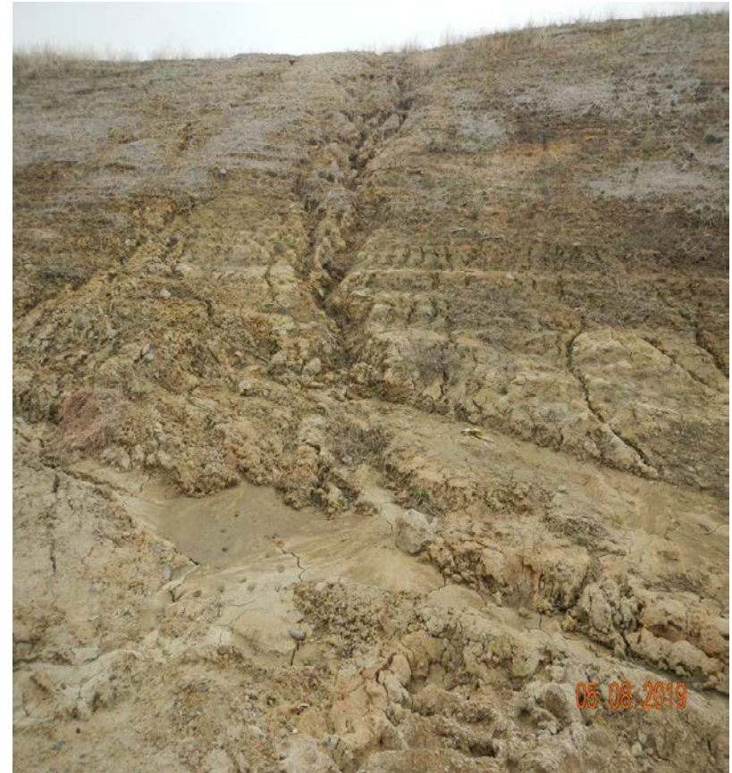
Photo#3: Erosion is occurring on SE corner of cut slope, sediment is migrating onto Location.
