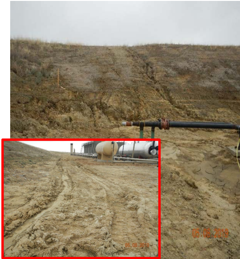
Photo#2: Erosion is occurring on SE corner of cut slope. Rutting behind equipment.
