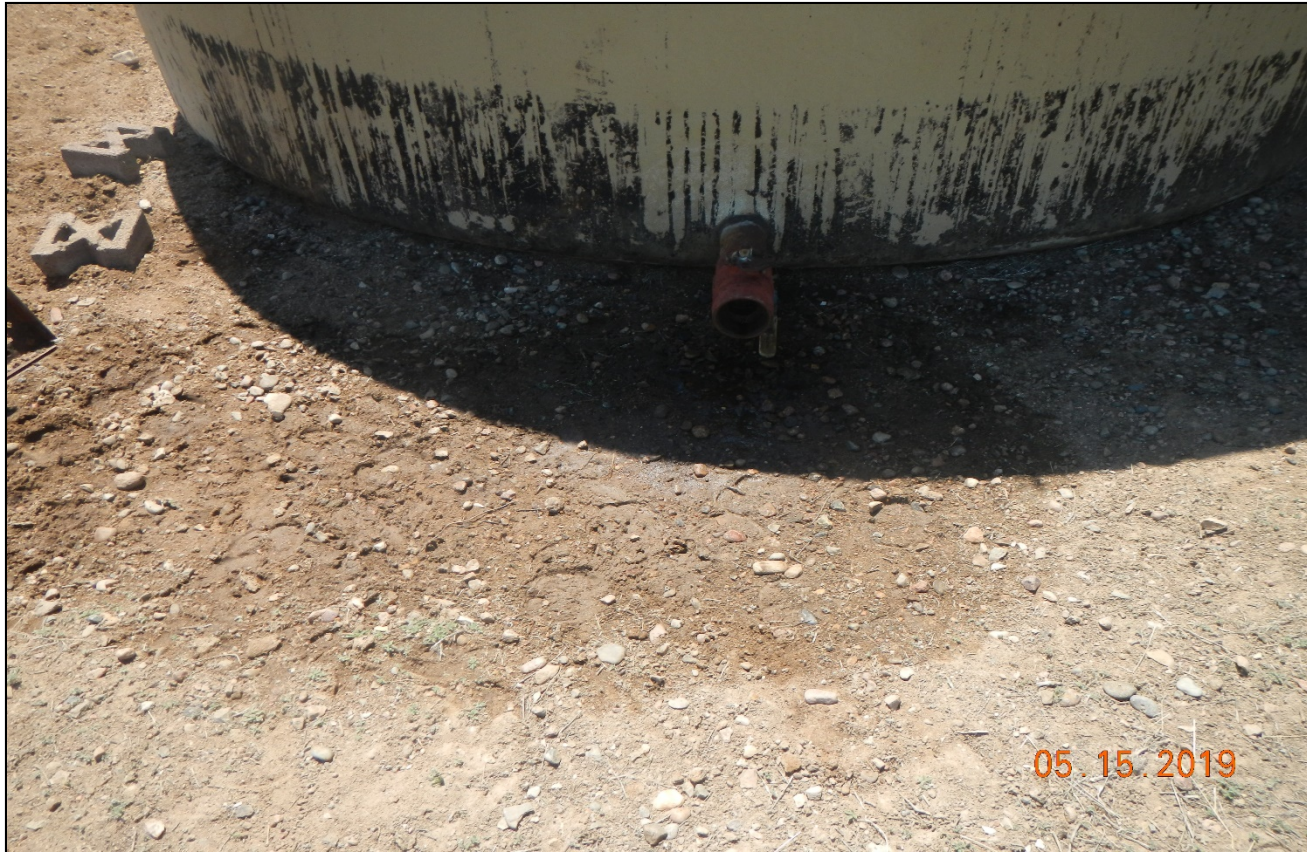
Photo 2. There was a dripping water leak coming from the condensate tank. Operator was notified the same day.
