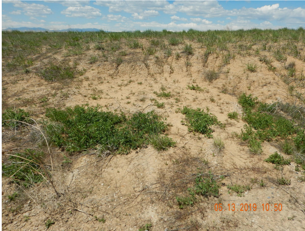
Photo 5. Photo taken from the southwestern location, facing West. Photo illustrates stormwater erosion. Operator has failed to properly stabilize cut slopes to minimize erosion and site degradation.
