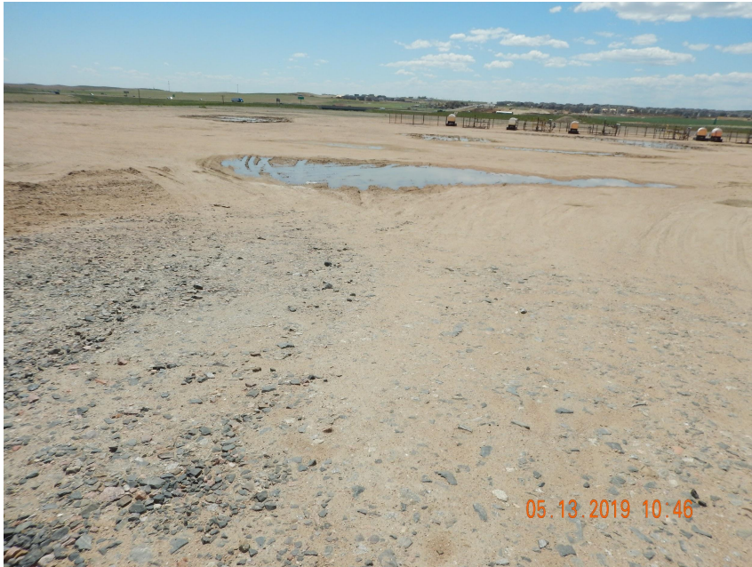
Photo 1. Photo taken from the entrance of location, facing Southeast. Photo illustrates that interim reclamation has not been performed. This location is not in compliance with Rule 1003 standards.
