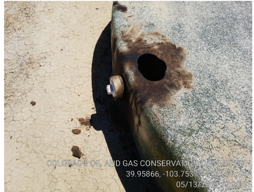
Pic 18 no netting on water tank.
