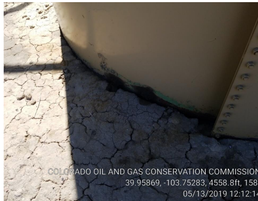
Pic 10 possible leak on tank
