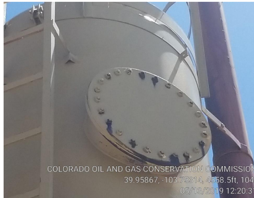
Pic 20 possible leak on separator
