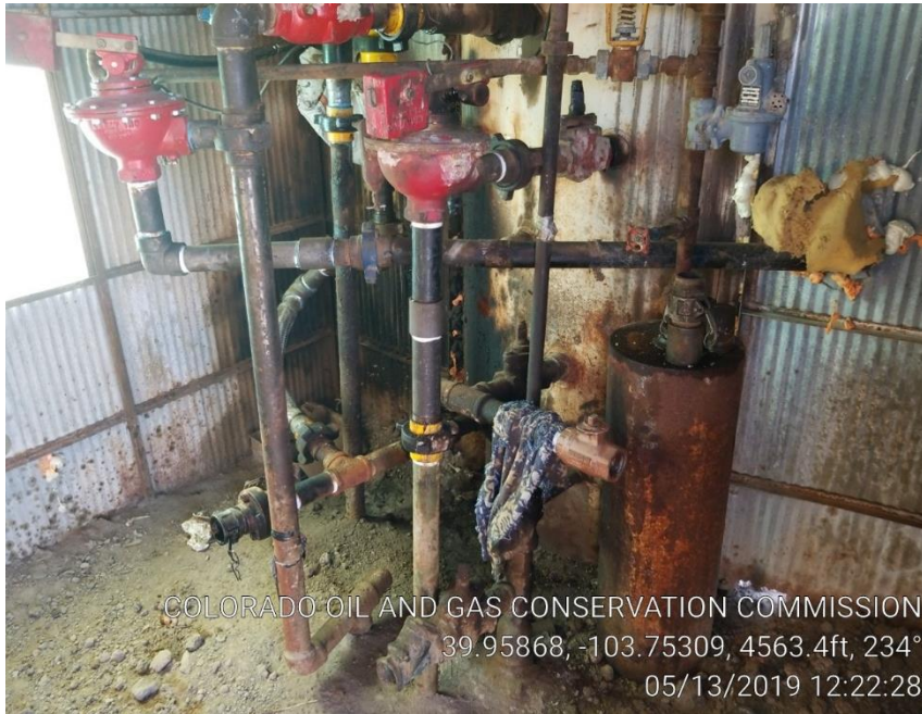
Pic 21 possible leak in separator house
