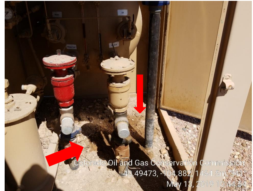
Photo 4: Stained soil inside east separator house.
