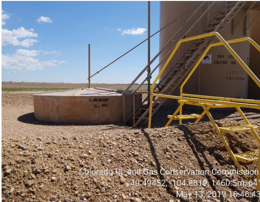
Photo 3: No NFPA placard on produced water tank.
