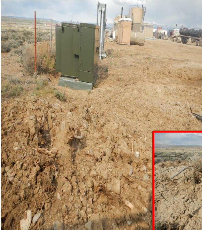
Photo#7: Stockpiles have no BMPs.
