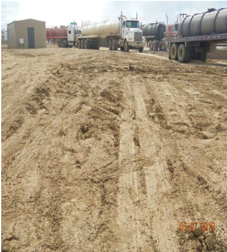
Photo#9: Rutting, sediment migration was observed.
