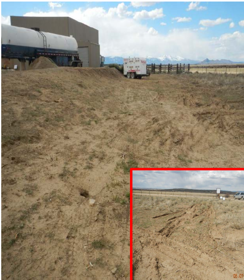
Photo#5: Perimeter BMPs/delineation is not apparent.
