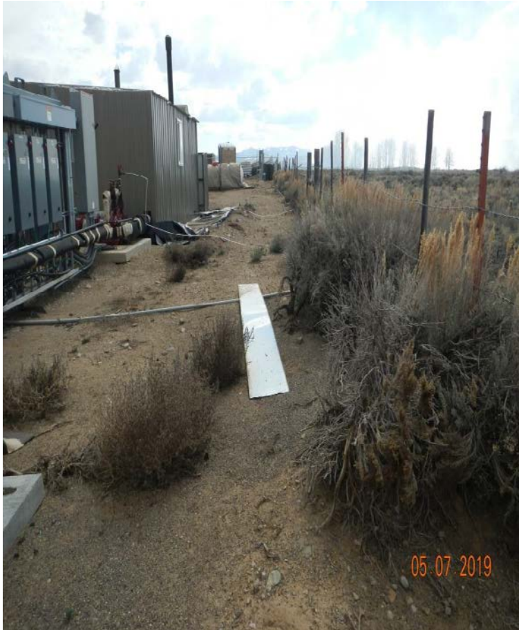
Photo#3: Perimeter BMPs/delineation is not apparent.
