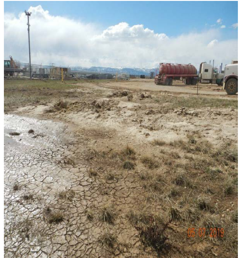
Photo#12: Lack of appropriate BMPs at South side of site.
