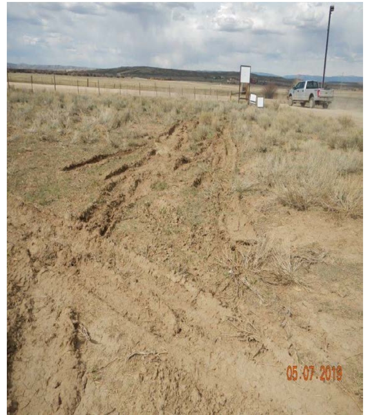
Photo#10: Rutting, sediment migration was observed.
