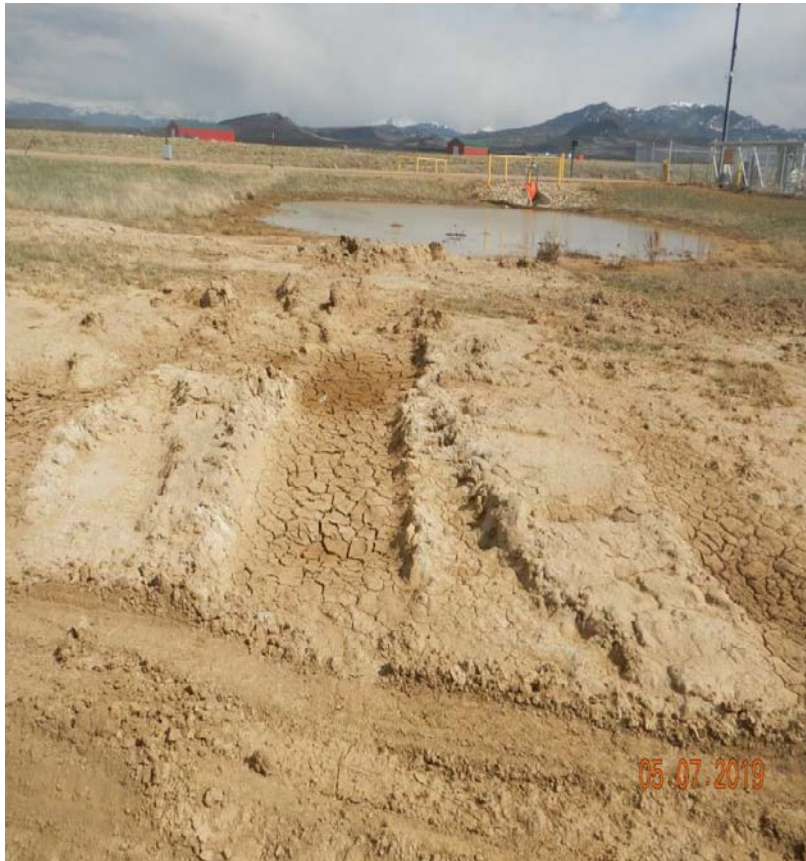
Photo#11: Lack of appropriate BMPs at South side of site.
