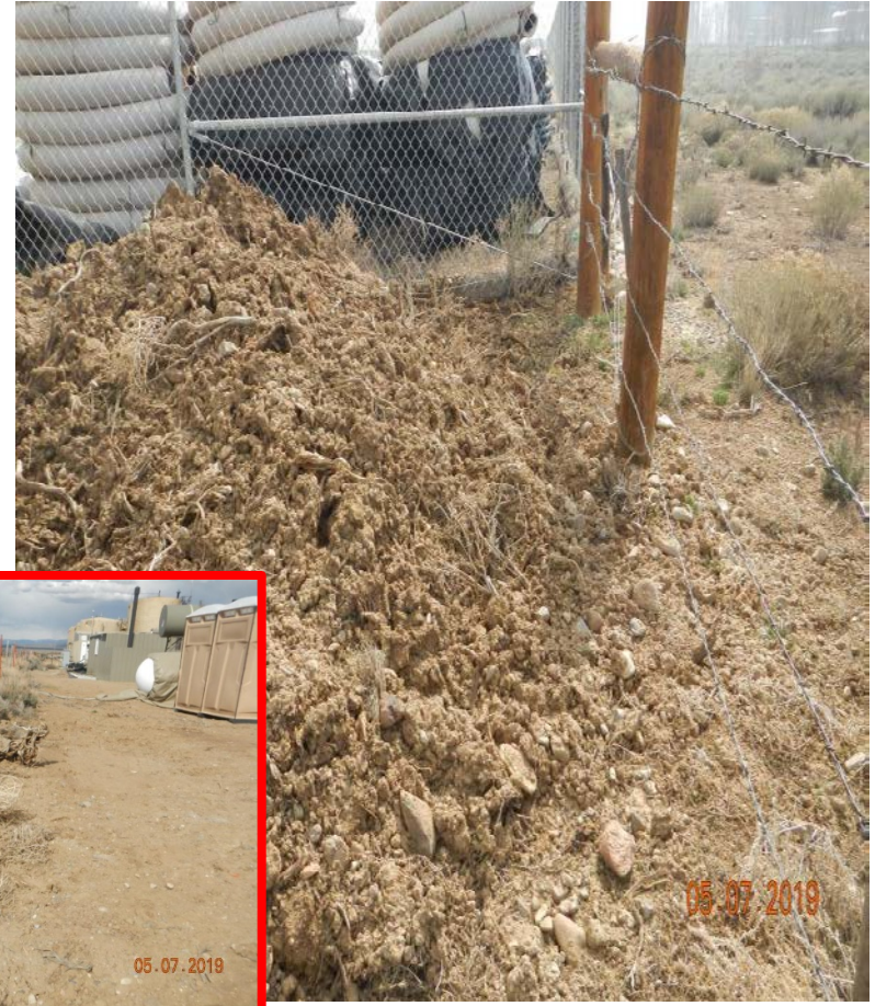
Photo#8: Stockpiles have no BMPs.
