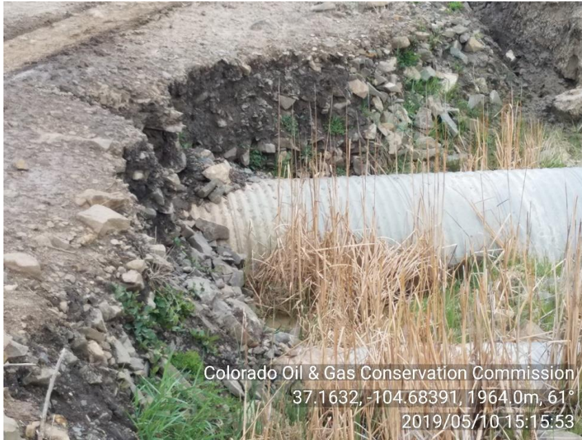
PHOTO 3: ROAD ACROSS STATE WATERS CROSSING IS ERODING ON SOUTH SIDE OF CROSSING. Install or repair required BMPs per Rule 1002.f.
