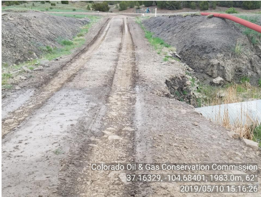
PHOTO 5: ANOTHER ANGLE OF EROSION FROM PHOTO #3.
