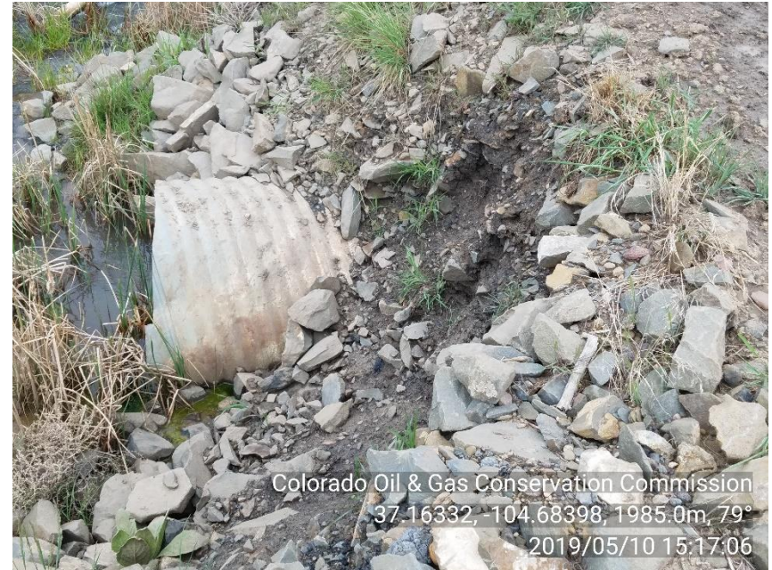
PHOTO 6: ROAD ACROSS STATE WATERS CROSSING IS ERODING ON NORTH SIDE OF CROSSING. Install or repair required BMPs per Rule 1002.f.
