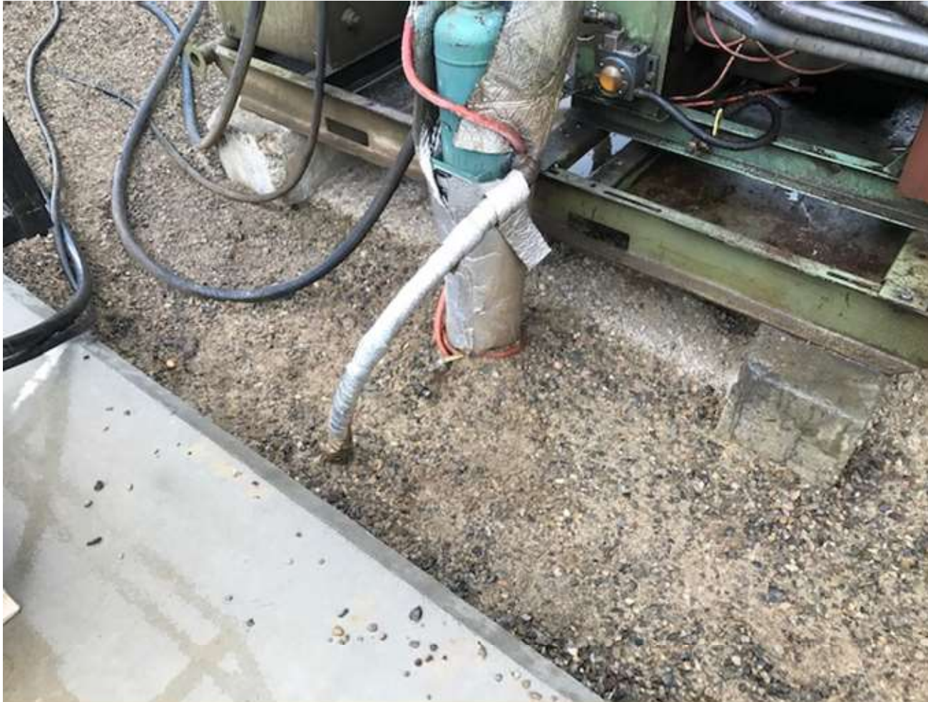
PHOTO 2: THE IMPACTED SOIL AROUND THE ENGINE SKID WAS REMOVED FROM THE LOCATION. (PHOTO TAKEN DURING RAIN SHOWERS).
