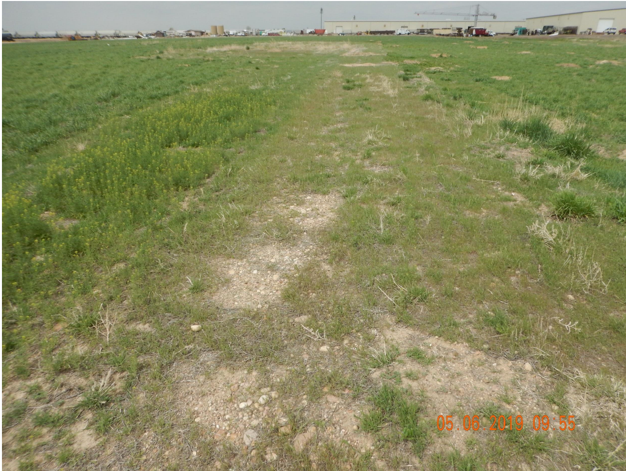
Photo 1. Photo taken from a portion of the access road, facing West. Access road is evident, with gravel, and has not been reclaimed per Rule 1004. It does not appear that the Operator has performed final reclamation activities throughout the access road and tank battery. Vegetation mainly consists of Cheatgrass and Kochia, all undesirable species. Reference area vegetation appears to be cropland, Winter wheat.
