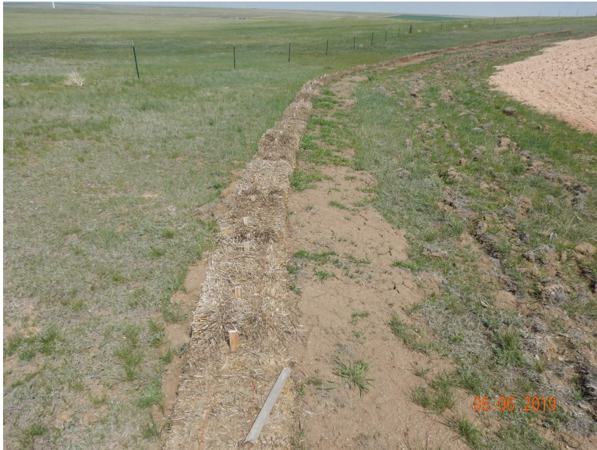
Photo 8: Photo taken from the west end of the location, facing north. Photo shows straw bale wattles. BMPs appear to be in proper functioning condition.
