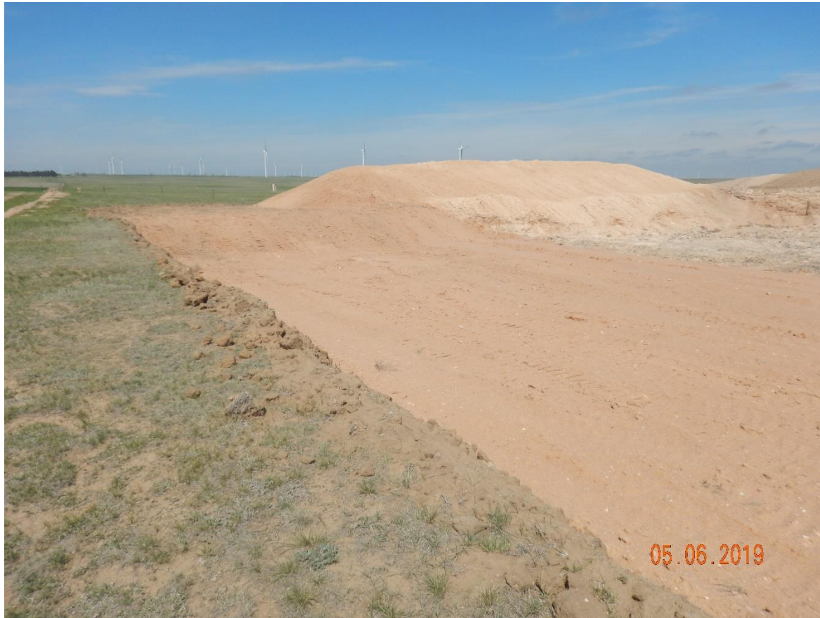
Photo 4: Photo taken from the south end of the location, facing west. Photos 4-7 provide an overview of the location from west, northwest, northeast to east. Photos shows interim reclamation activities do not yet appear to have been conducted on the location.
