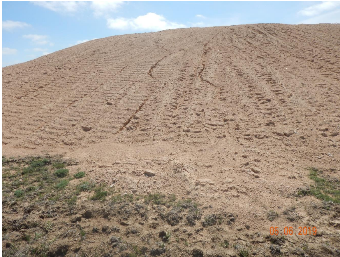
Photo 9: Photo taken from the west end of the location, facing east. Photo shows erosion degradation occurring on slopes of the soil stockpile and sediment deposition.
