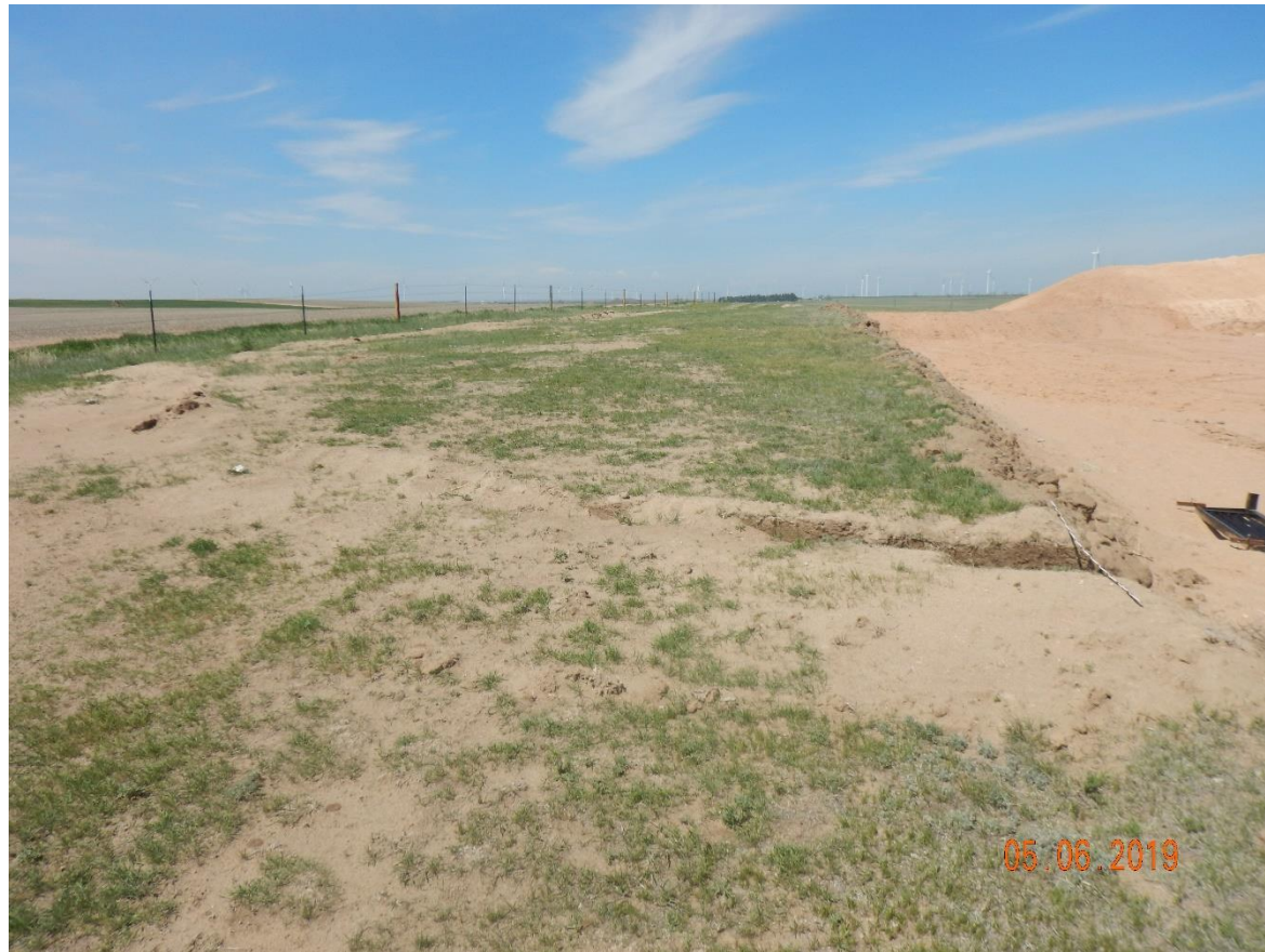
Photo 2: Photo taken from the south end of the location, facing west. Photo shows erosion degradation occurring on the south end of the location. 6 foot measuring stick for reference.
