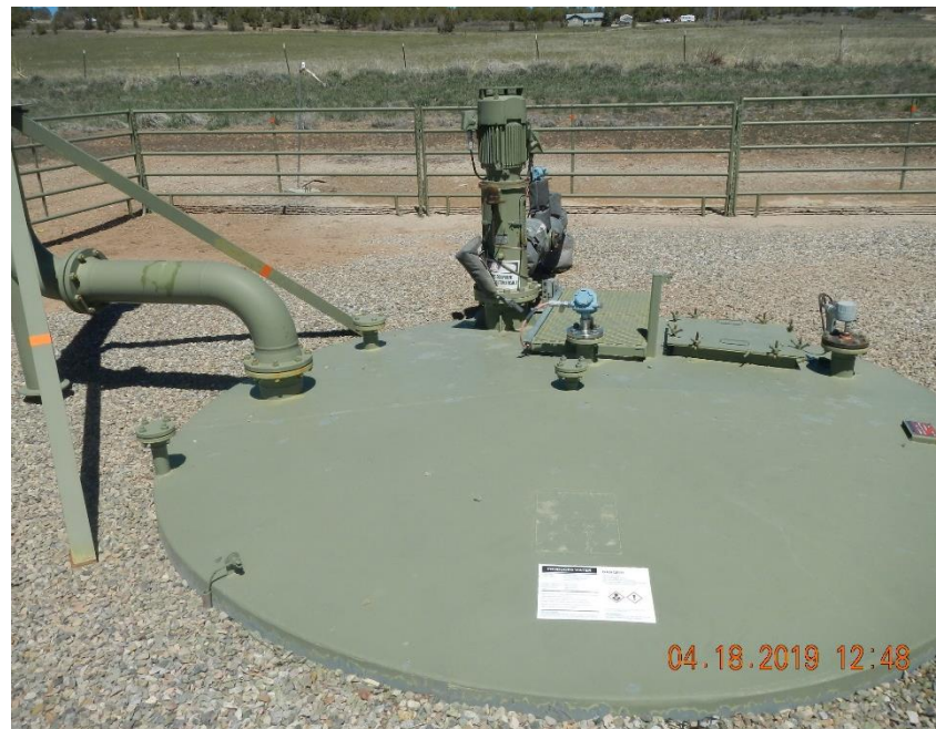
Double walled steel PBV.
