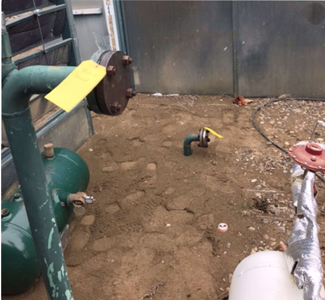
PHOTO 3: THE ABOVE GROUND PIPES ARE FLANGED AND MARKED.
