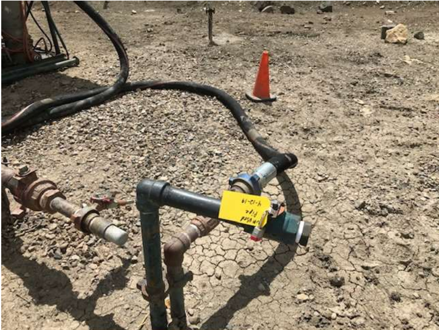
PHOTO 2: THE RISERS WERE LOTO AND MARKED.
