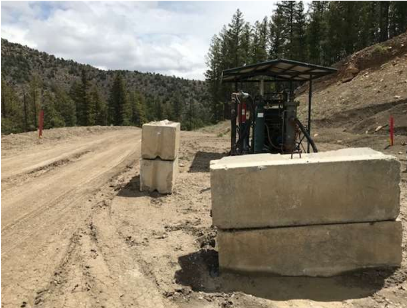
PHOTO 4: THE CEMENT BLOCKS WERE USED TO PROTECT THE WELL HEAD FROM TRAFFIC. THE BLOCKS WERE PLACED BACK AROUND THE WELL HEAD.
