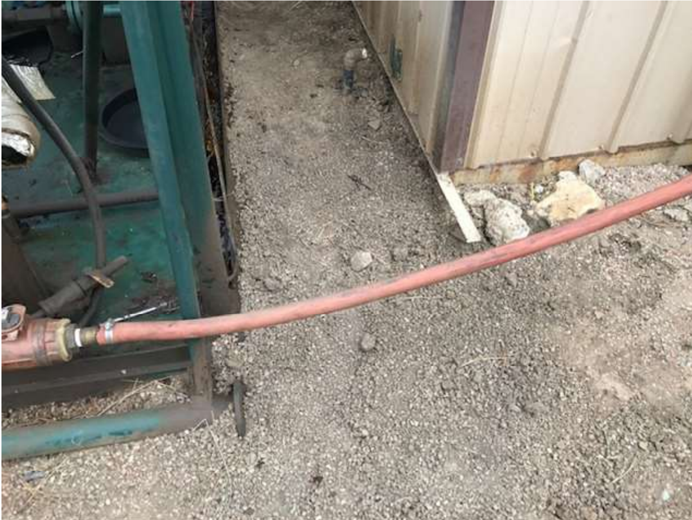
PHOTO 1: THE IMPACTED SOIL AROUND THE LIQUID RING COMPRESSOR WAS REMOVED FROM THE LOCATION. THE COMPRESSOR SKID WAS CLEANED UP.
