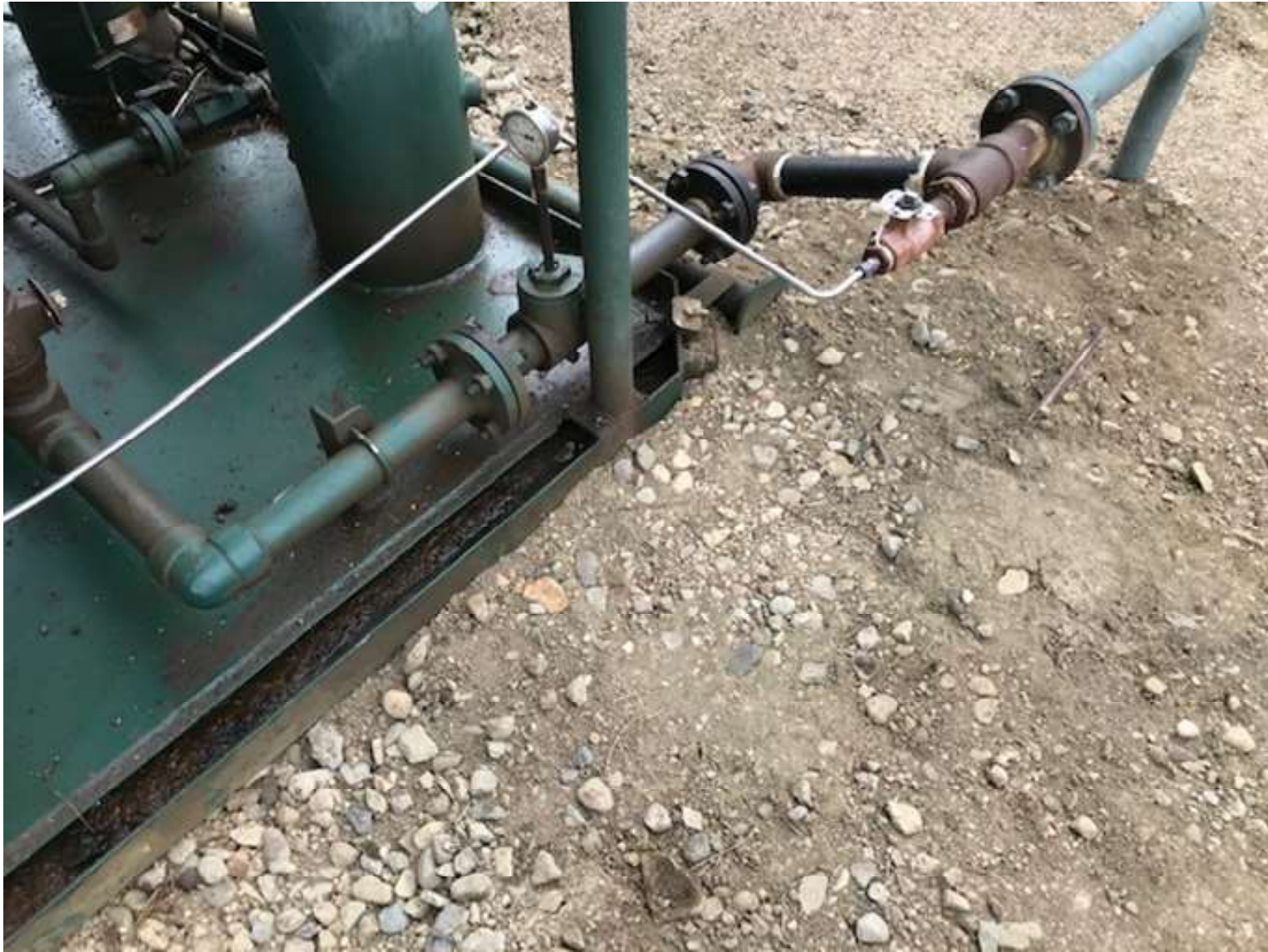
PHOTO 3: THE FLUID ACCUMULATION WAS REMOVED FROM THE RESERVOIR. THE IMPACTED SOIL AROUND THE LIQUID RING COMPRESSOR WAS REMOVED FROM THE LOCATION.
