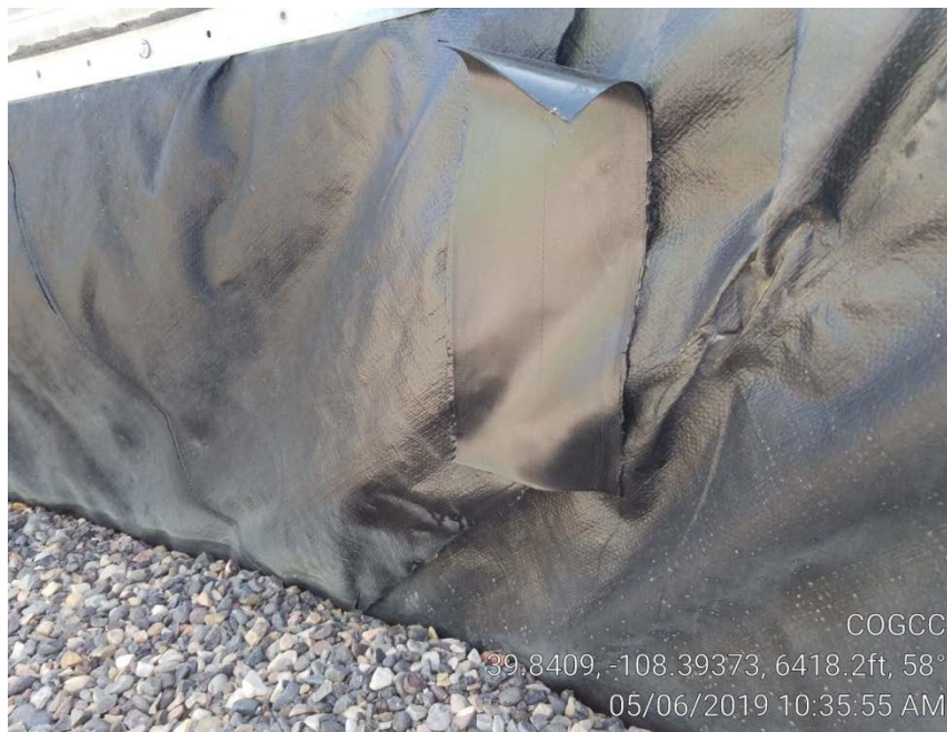
Photo 2. Liner repair inadequate.
