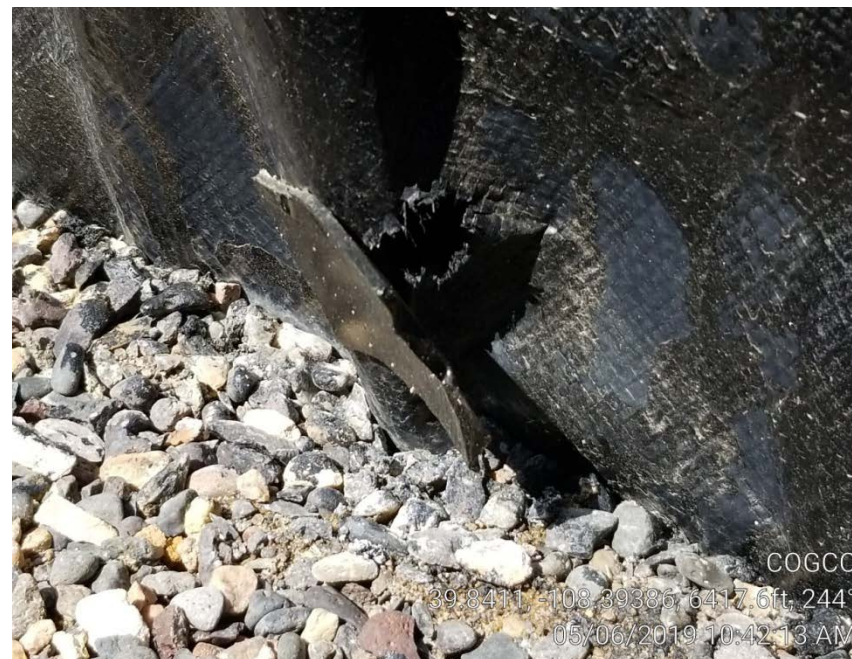
Photo 3. Liner repair inadequate.
