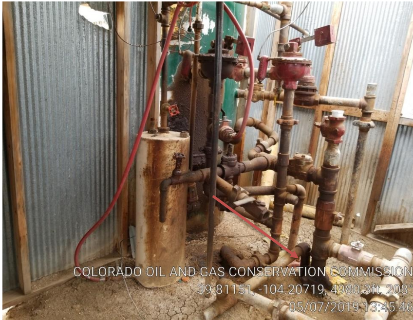
Pic 9 possible leak separator house stained soil
