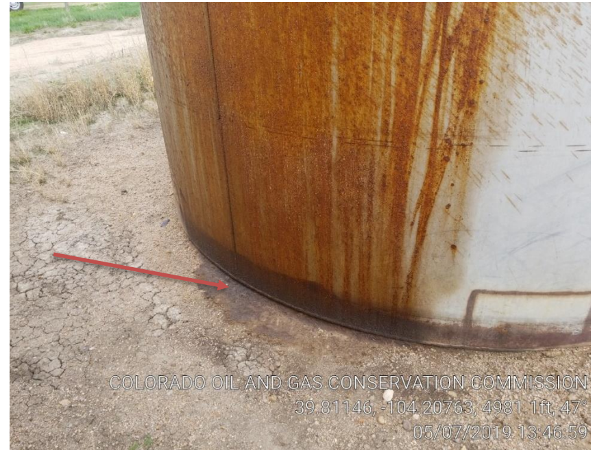
Pic 12 stained soil overflowing tank
