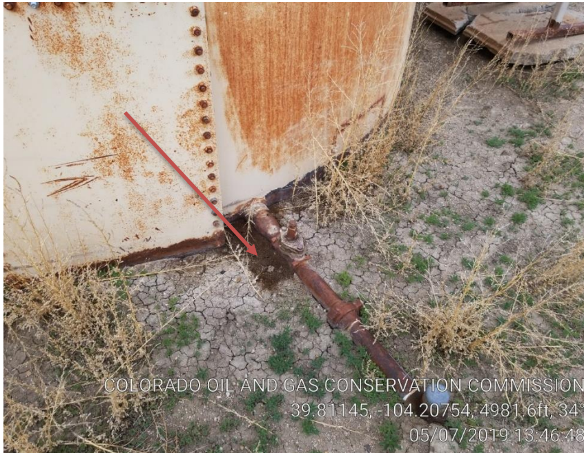
Pic 11 stained soil possible leak
