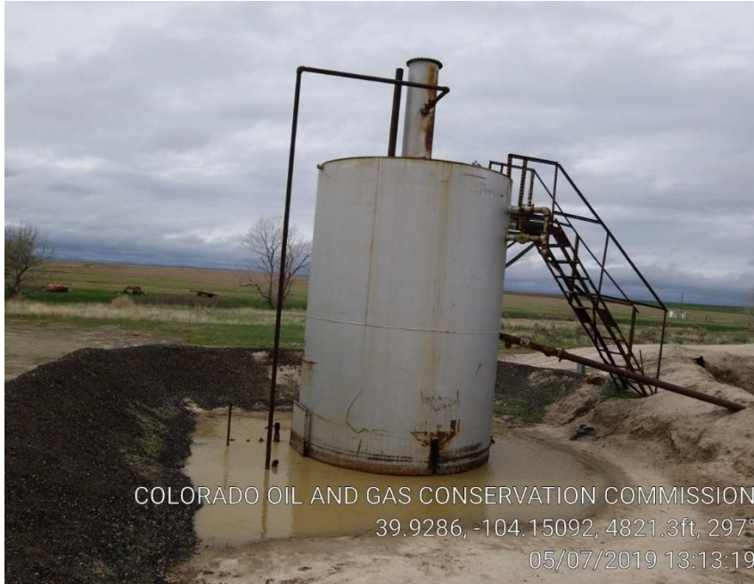
Pic 7 water pooled in water tank containment, possible leak.
