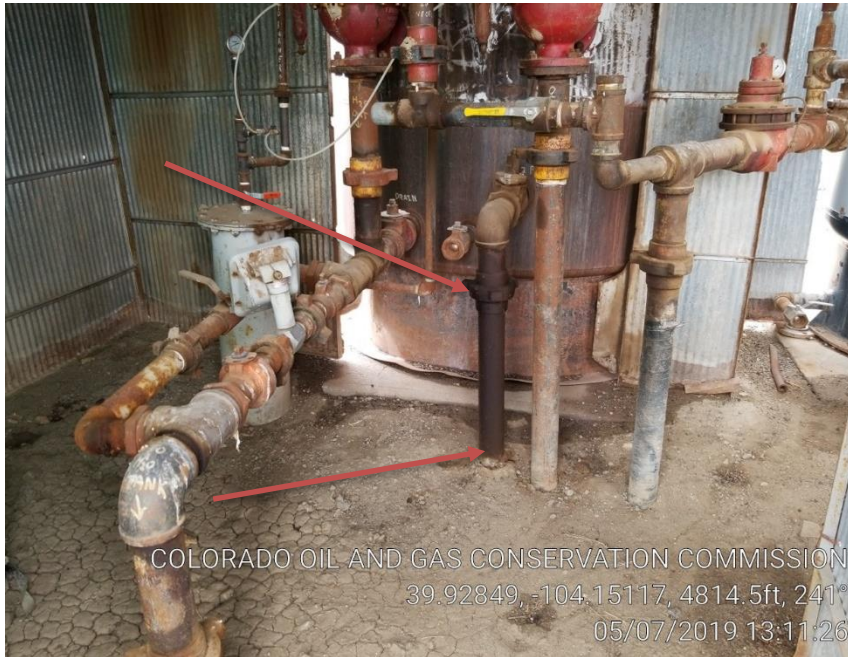
Pic 5 stained soil possible leak.
