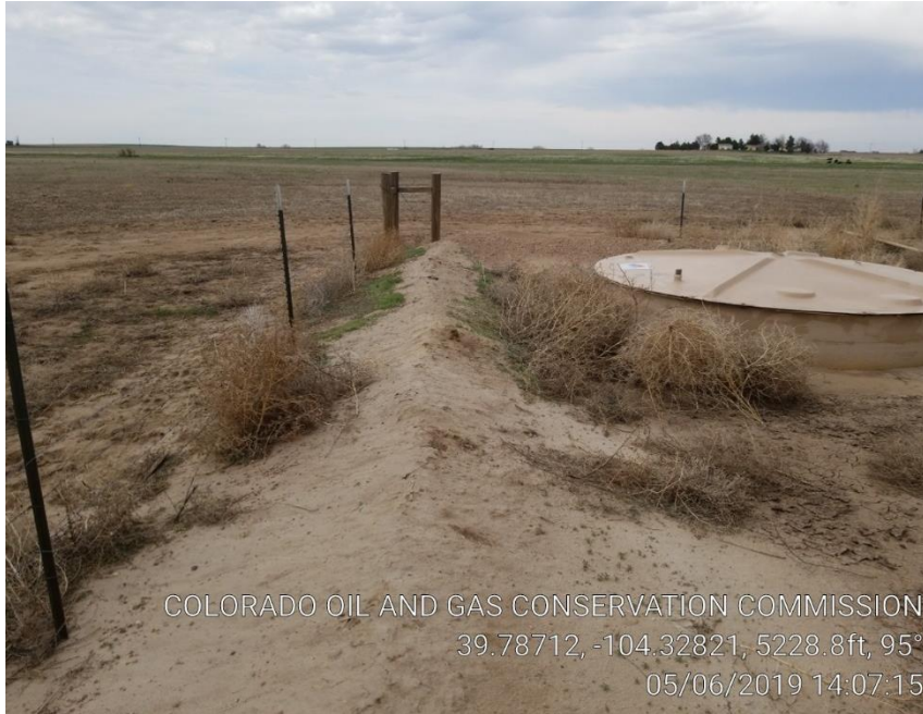
Pic 11 inadequate berm. Weeds.
