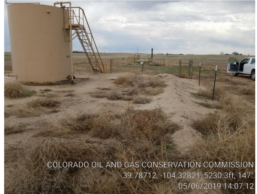
Pic 10 weeds, inadequate berm
