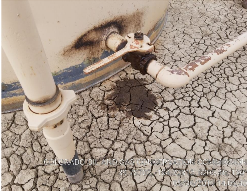
Pic 9 stained soil possible leak
