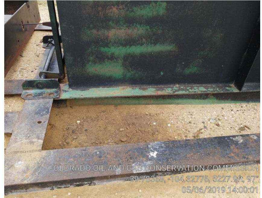
Pic 2 stained soil possible leak
