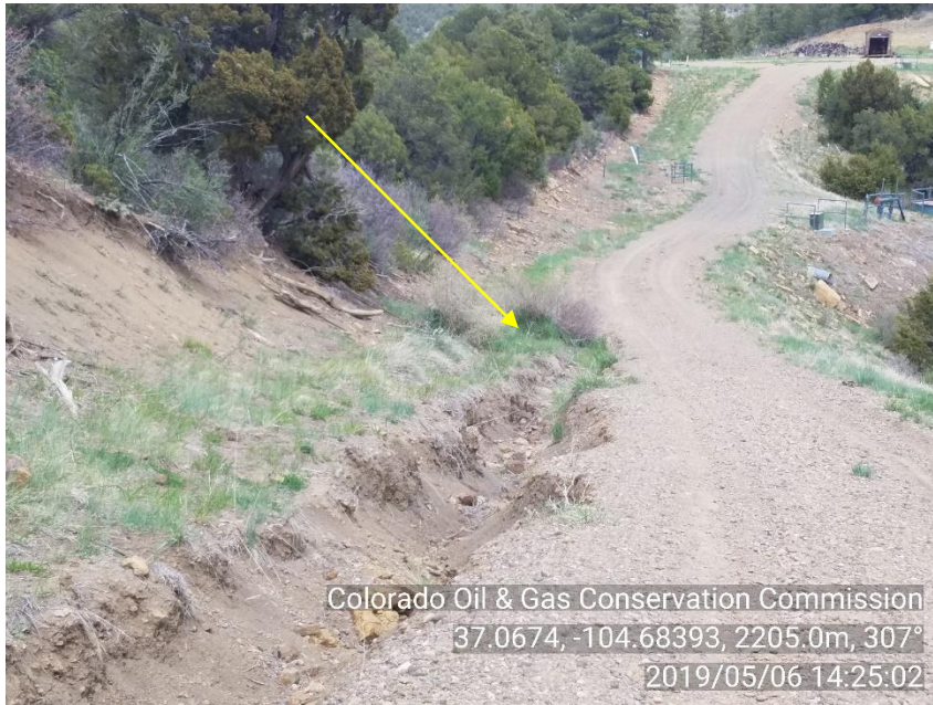
PHOTO 5: IMAGE SHOWING THE START OF SEDIMENT DEPOSITS FILLING STORMWATER DRAIN.
