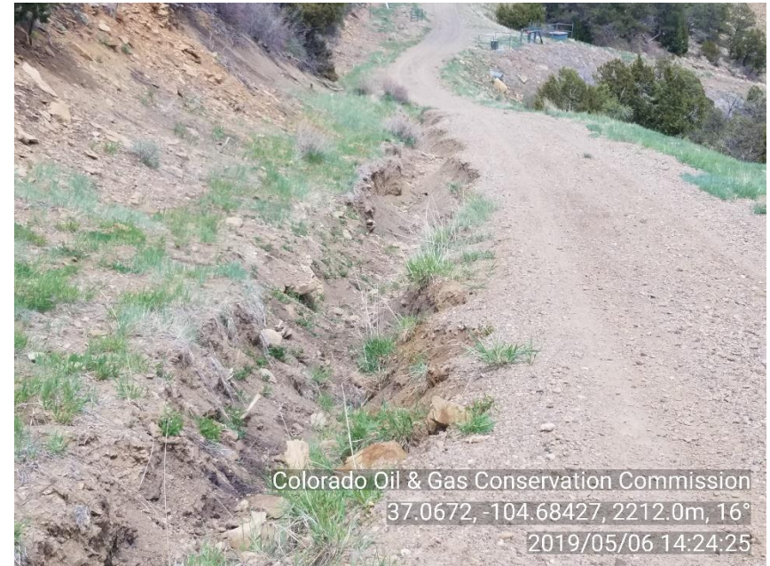
PHOTO 4: BMP FAILURE APPROXIMATELY 25 YARD DOWNSLOPE FROM CREST OF SLOPE.
