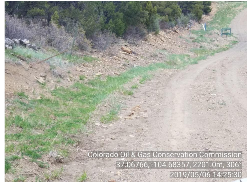
PHOTO 6: STORMWATER DRAIN FILLED WITH SEDIMENT NEAR THE BOTTOM OF THE SLOPE.
