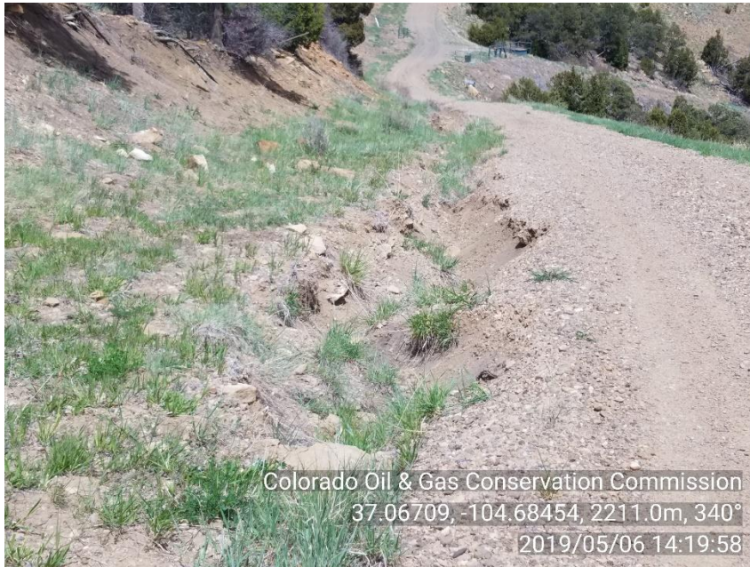
PHOTO 3: STORMWATER DRAINAGE DITCH ON UPSLOPE SIDE OF ROW WEST OF LOCATION IS WASHED OUT. Install or repair required BMPs per Rule 1002.f.
