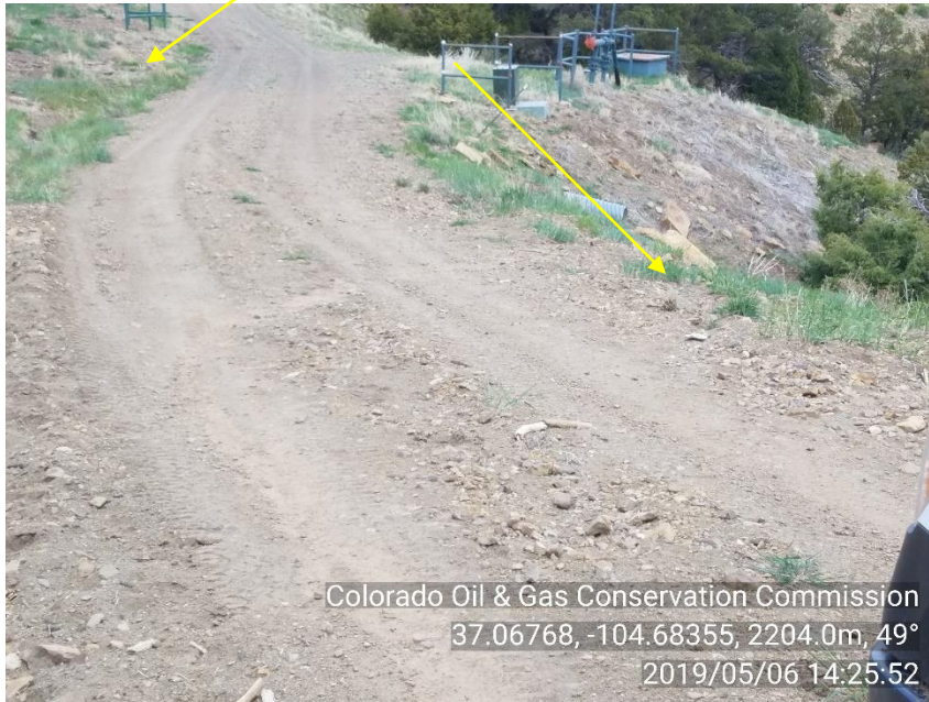
PHOTO 7: IMAGE SHOWING STORMWATER CROSSING ROAD APPROXIMATELY 10 TO 15 YARD BEFORE THE CULVERT UPPER ARROW SHOWS THE MOUTH OF THE CULVERT THE ARROW ON THE RIGHT SHOWS WHERE STORMWATER IS RUNNING ACROSS ROW.
