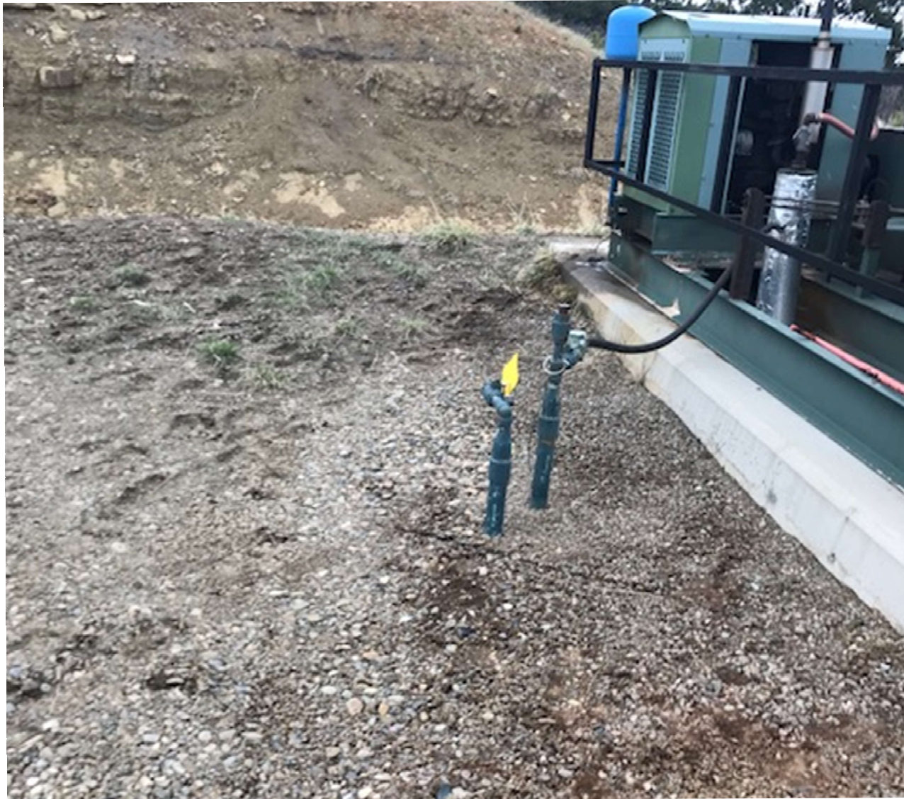
PHOTO 3: UNUSED RISERS WERE LOTO AND MARKED.
