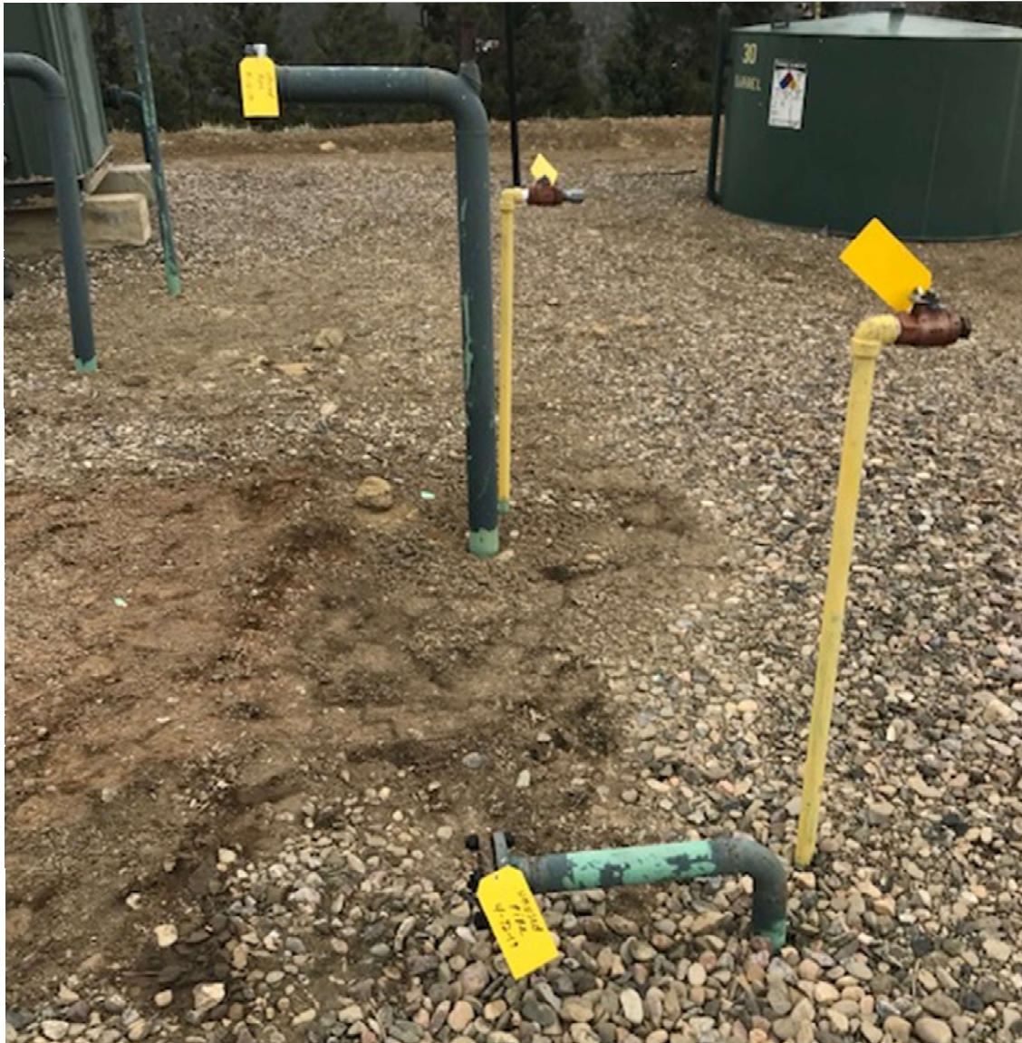
PHOTO 2: UNUSED RISERS WERE LOTO AND MARKED.
