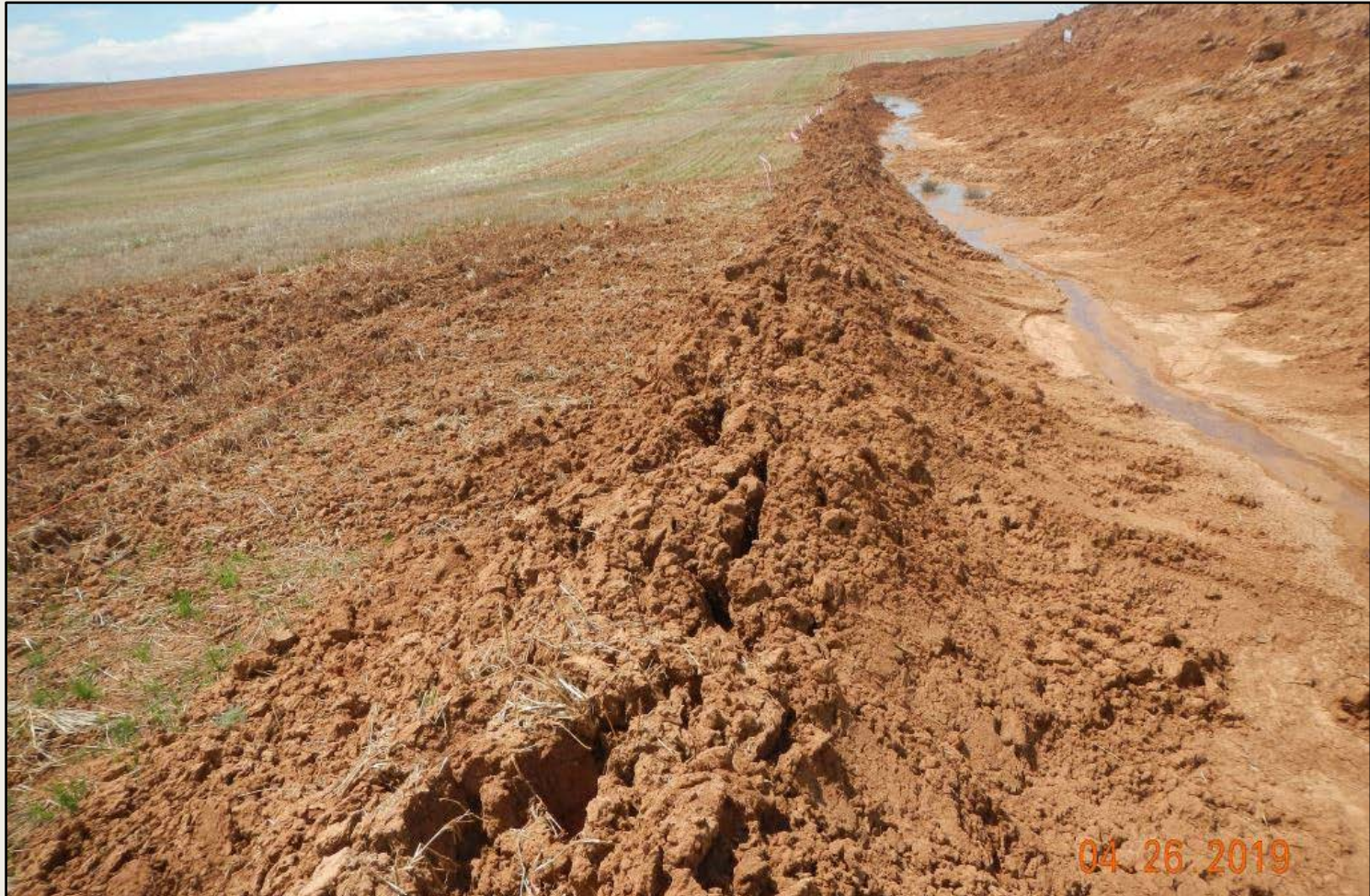
Photo 1. View of the southern project area from the southeastern corner facing westward. Loose soils present around the perimeter of the project area will rapidly erode.
