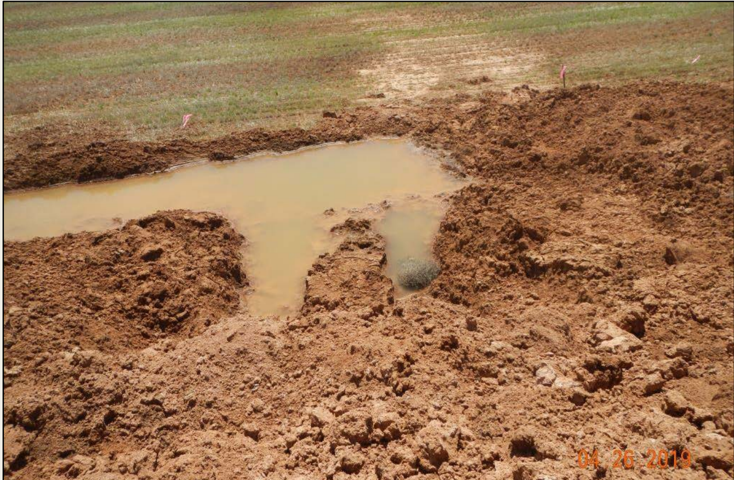
Photo 3. View of a silt trap in the southwestern project area. Silt trap is not properly sized or stabilized, and outlet is not present. Evidence of overflow observed.
