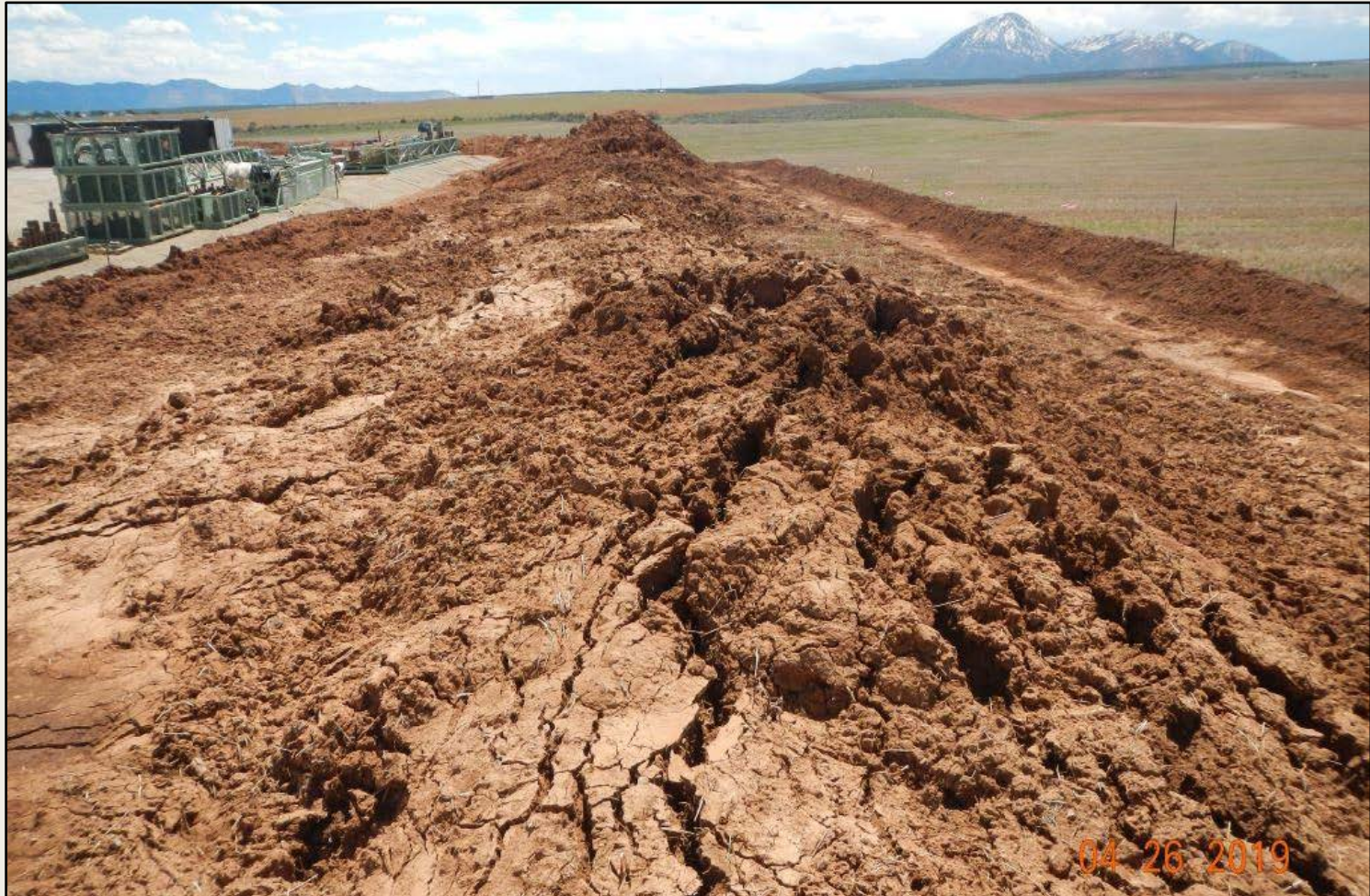
Photo 4. View of the western project area from the northwestern edge facing southward. Exposed soils are loose and eroding. Loose perimeter soil present.
