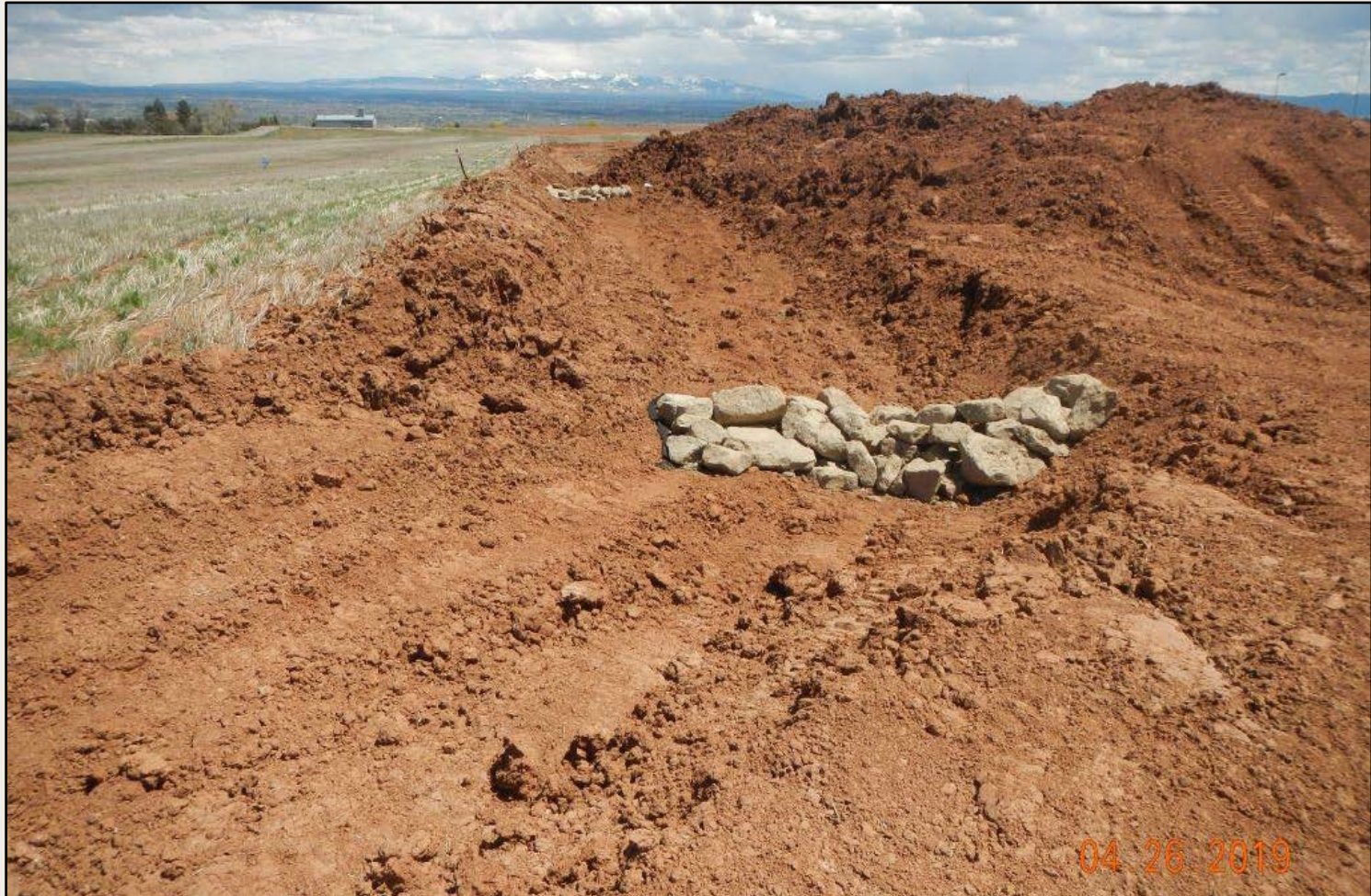
Photo 5. View of check dams along northeastern edge of the project area. Exposed soil will rapidly erode into ditches.
