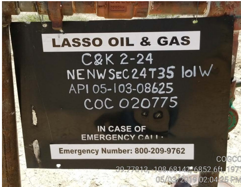
Photo 2. Well head sign missing nearest public road and "911".
