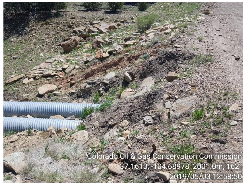
PHOTO 4: STORMWATER EROSION AT CULVERT NORTH OF LOCATION ON MAIN ROW.
