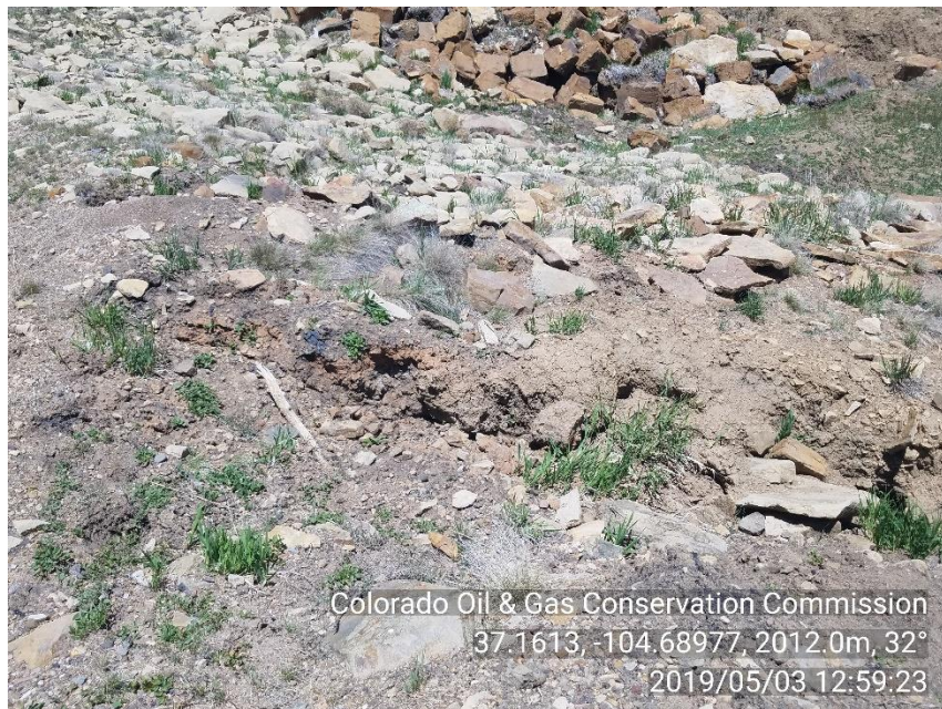
PHOTO 5: STORMWATER EROSION AT CULVERT NORTH OF LOCATION ON MAIN ROW.
