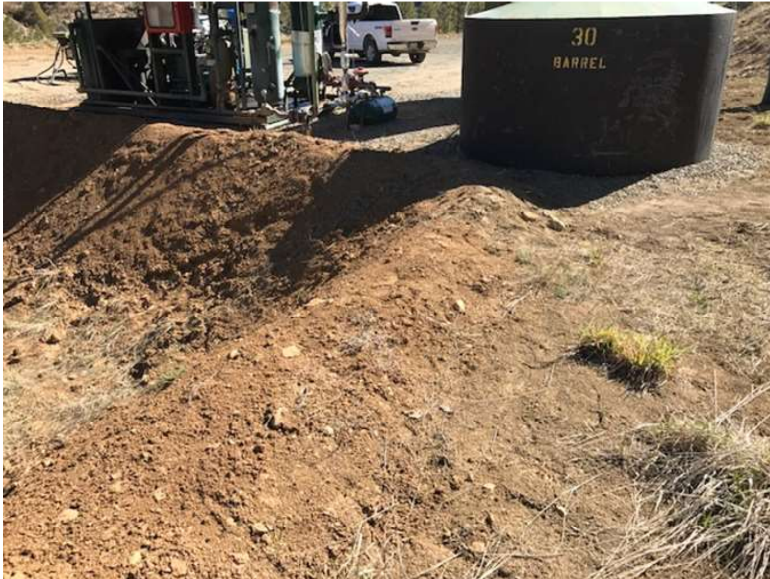
PHOTO 8: THE DIRT BERM WAS DOMINATED AND THE EROSION RILL CORRECTED.
