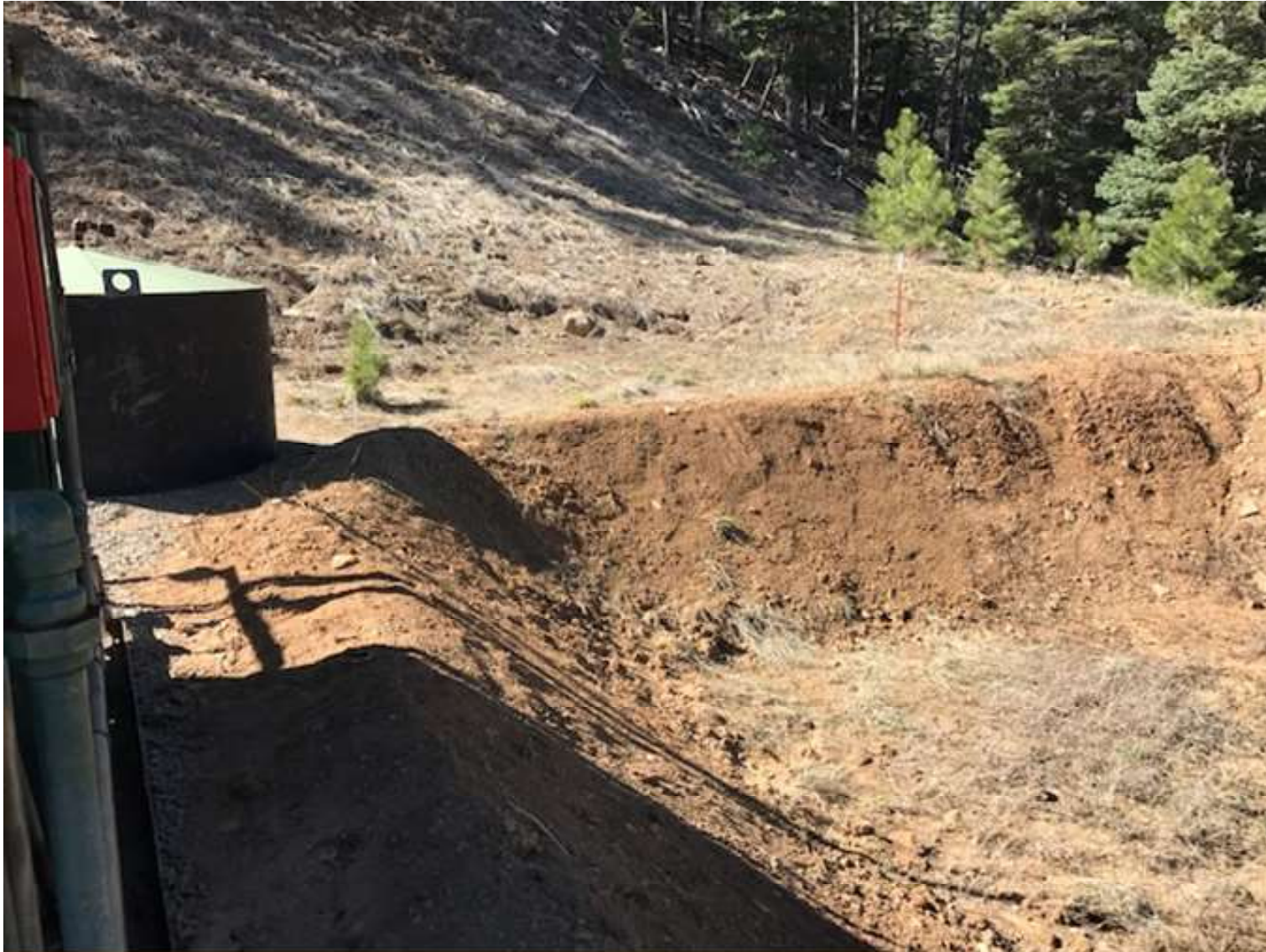
PHOTO 7: THE DIRT BERM WAS DOMINATED AND THE EROSION RILL CORRECTED.
