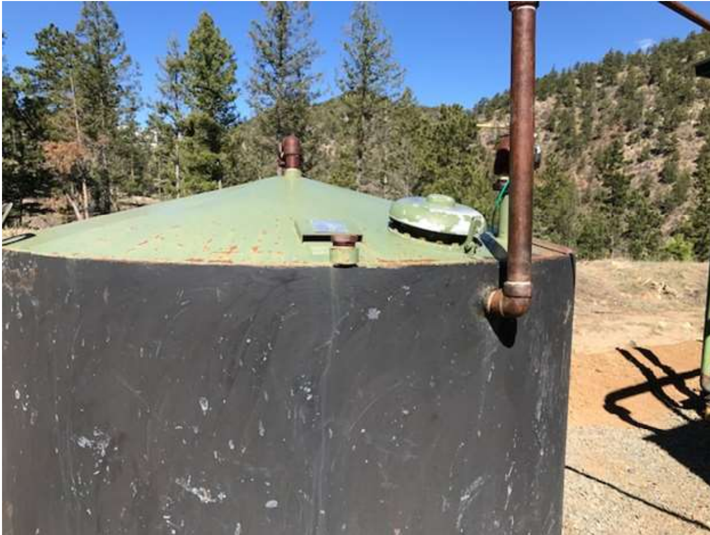
PHOTO 5: THE GAUGE HATCH WAS CLOSED IN ACCORDANCE WITH RULE 605.A .
