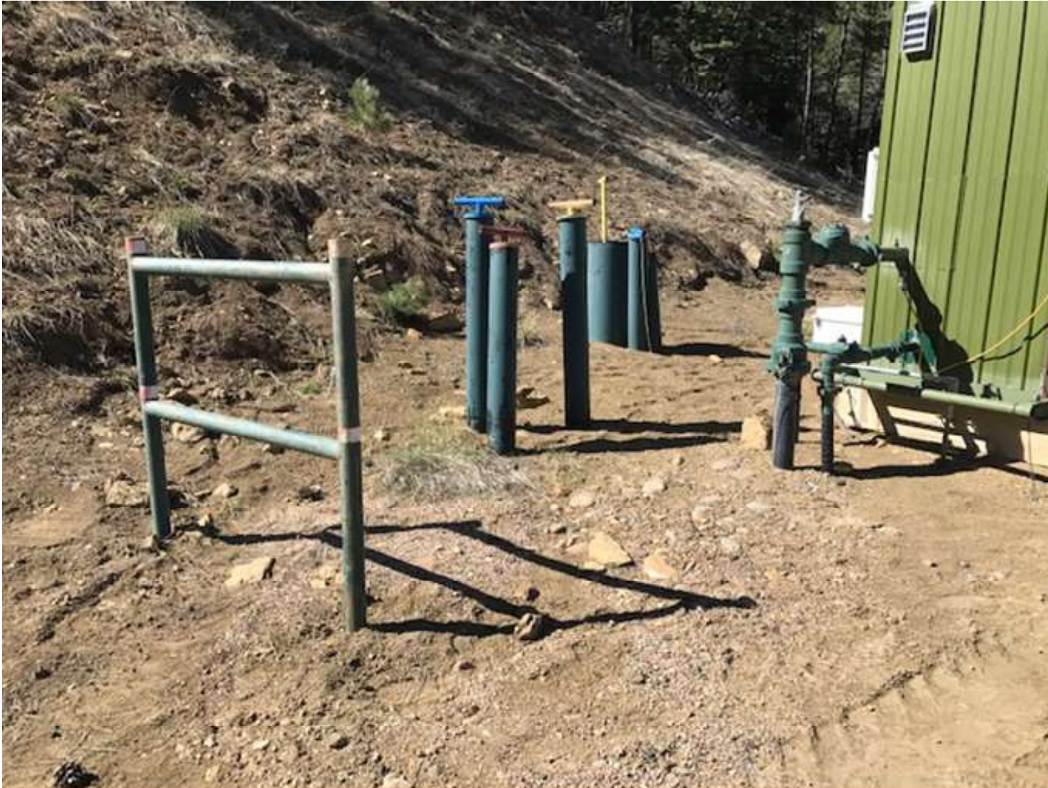
PHOTO 6: THE "H" BRACE GUARD WAS RE-INSTALLED IN FRONT OF THE VALVES TO PROTECT THE VALVES. THE RED "T" HANDLE WAS PLACED BACK ON THE VALVE.
