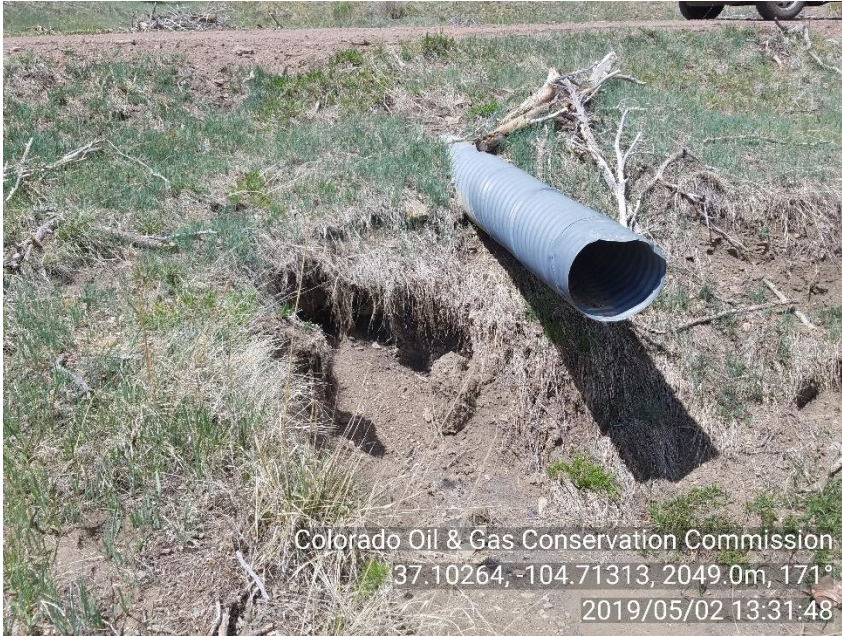
PHOTO 5: EROSION NEAR CULVERT OUTLET ON DOWN GRADIENT SIDE OF CULVERT.
