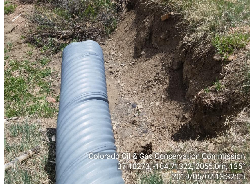
PHOTO 6: ANOTHER ANGLE OF EROSION ON DOWN GRADIENT SIDE OF CULVERT
