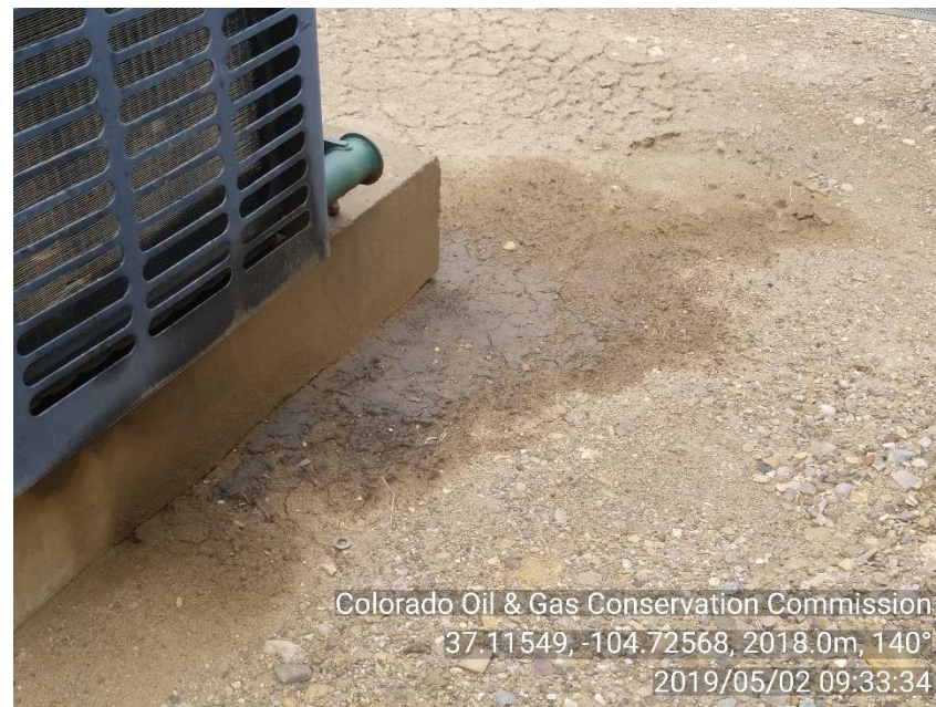
PHOTO 4: APPROXIMATELY 2' BY 3' AREA OF IMPACTED SOIL NEAR NORTHEAST SIDE OF PRIME MOVER ENGINE SKID.
