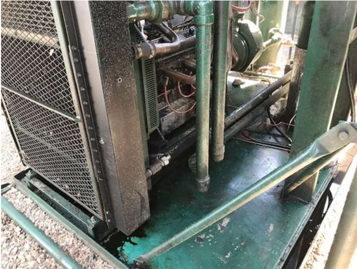
PHOTO 1: THE ABSORBENT PADS THAT WERE ON THE SKID WERE REMOVED AND THE OIL ACCUMULATION WAS CLEANED UP.
