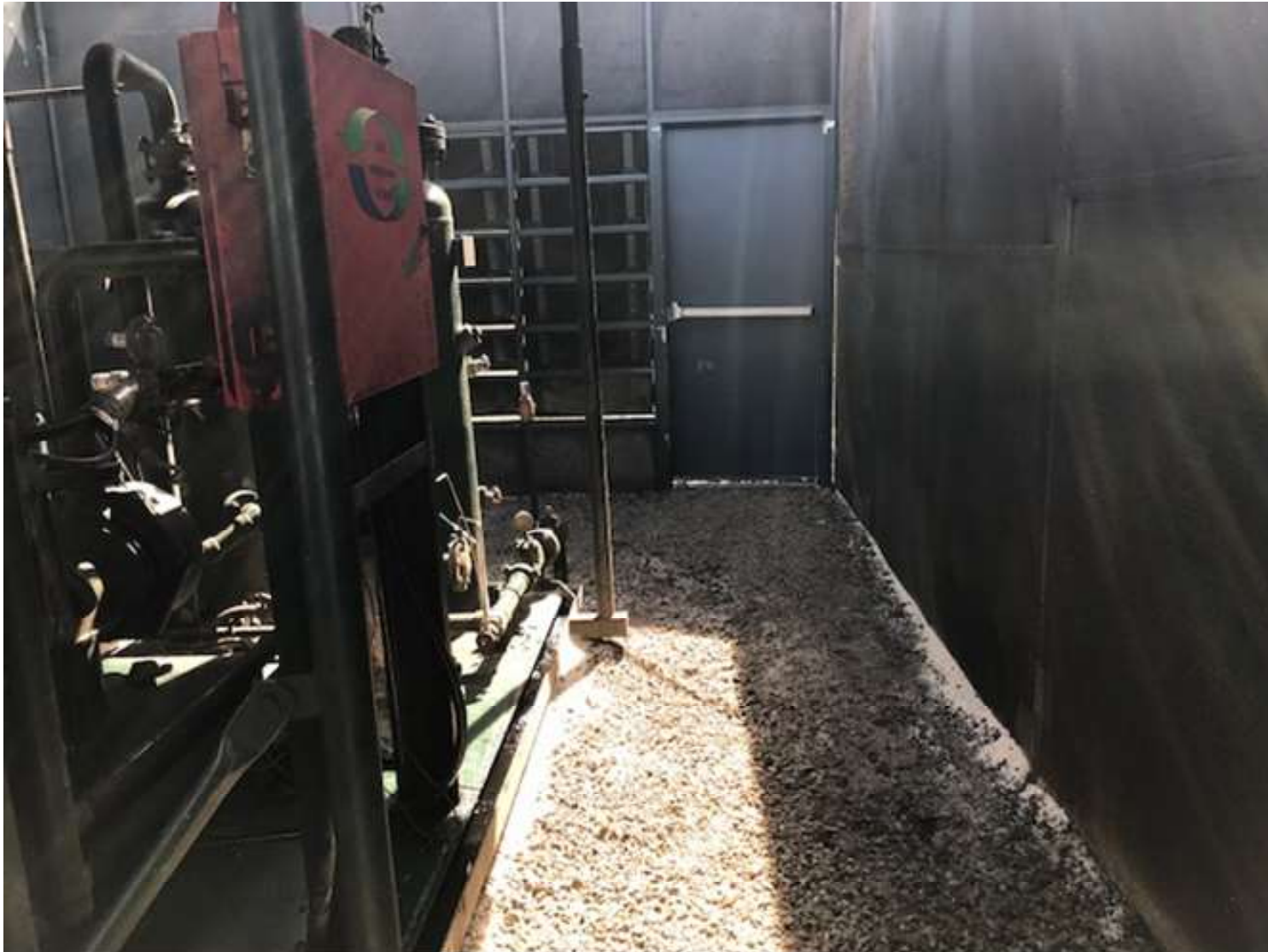
PHOTO 2: THE IMPACTED SOIL NEXT TO THE LIQUID RING COMPRESSOR AND THE SOUND WALLS HAVE BEEN CLEANED UP.
