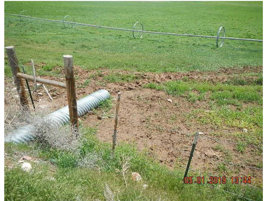
Lease Road discharge culvert
