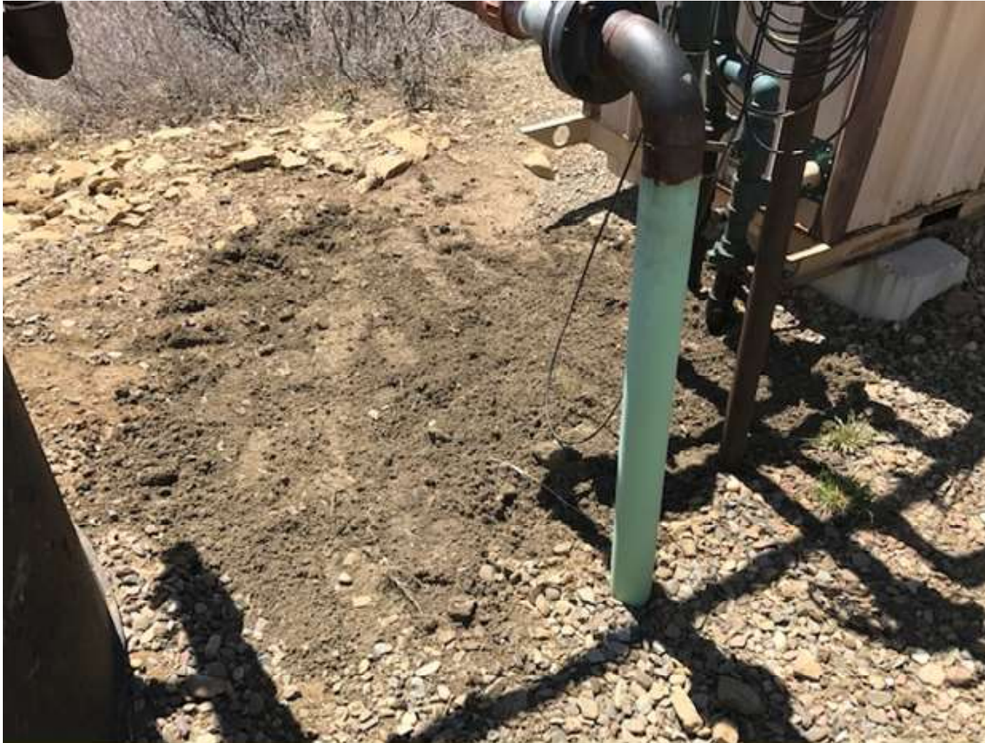
PHOTO 2: THE IMPACTED SOIL BEHIND THE SEPARATOR HOUSE WAS REMOVED FROM THE LOCATION.
