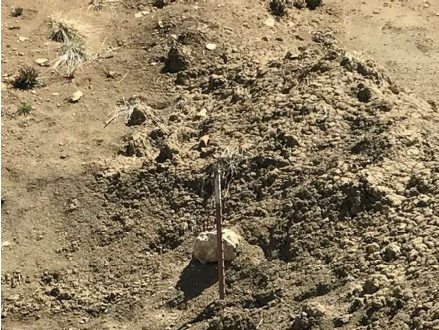
PHOTO 4: A RED POST WAS INSTALLED IN THE PRODUCTION PIT TO MARK THE TWO FOOT FREE BOARD LEVEL IN THE PIT.
